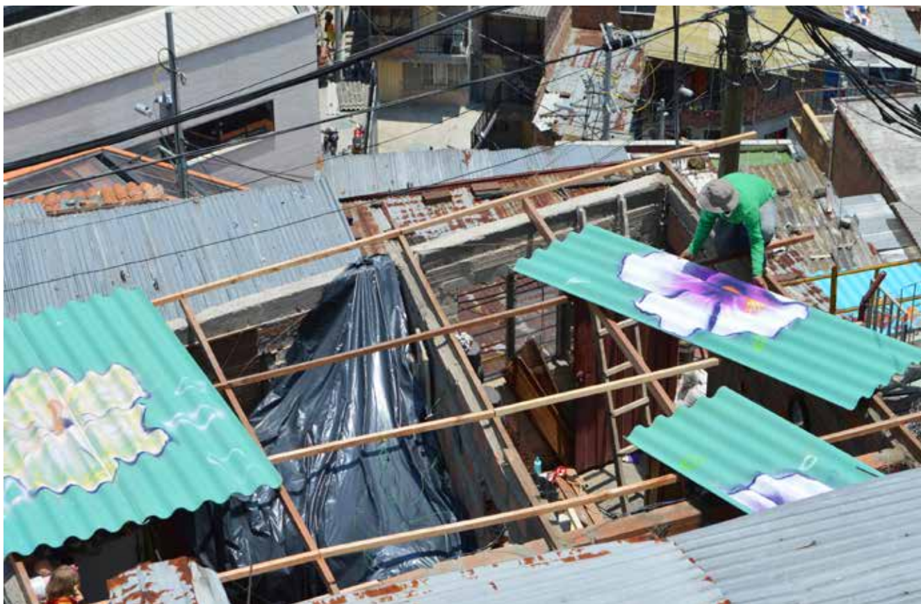
A local artist installs a newly painted roof in Medellín, Colombia © UN-Habitat/Julius Mwelu
