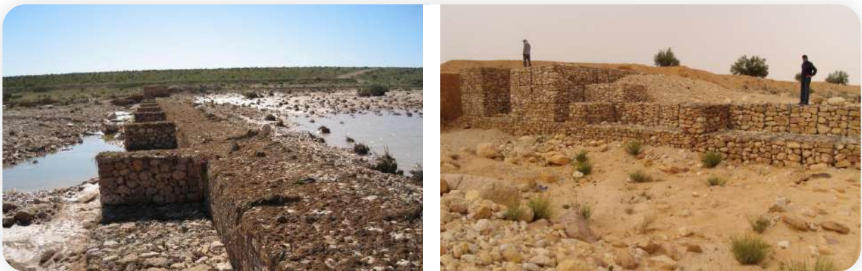
Figure 15 Gabion Check Dams
