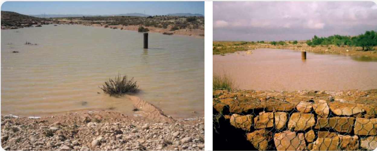
Figure 24 Recharge Well behind a Gabion Check Dam
