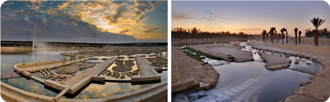
Figure 50 Water Filtration Facility, Wadi Hanifa, Riyadh, Saudi Arabia
