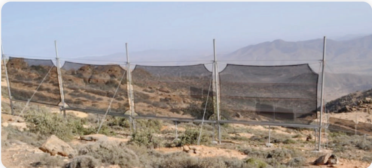
Figure 6 Dar Si Hmad's Phase 1 fogwater harvesting system includes 600 square meters of fog nets
