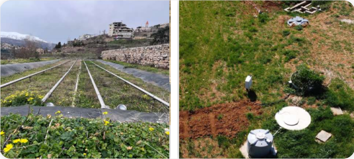
Figure 37 Decentralized Wastewater Treatment Systems (DEWATS) in Lebanon
