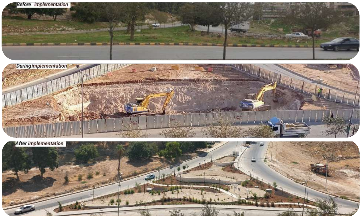
Figure 44 Construction Phases of the Al Zohour Green Triangle
