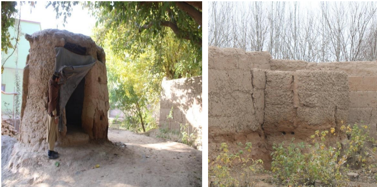
Bathrooms in poor and unhygienic conditions in the settlement.
