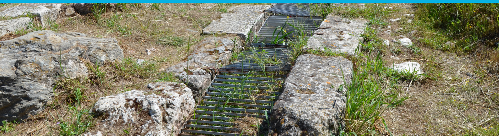
Section of the Hadrian Aqueduct near the ancient Agora, Athens. Photo: Carole Raddato
