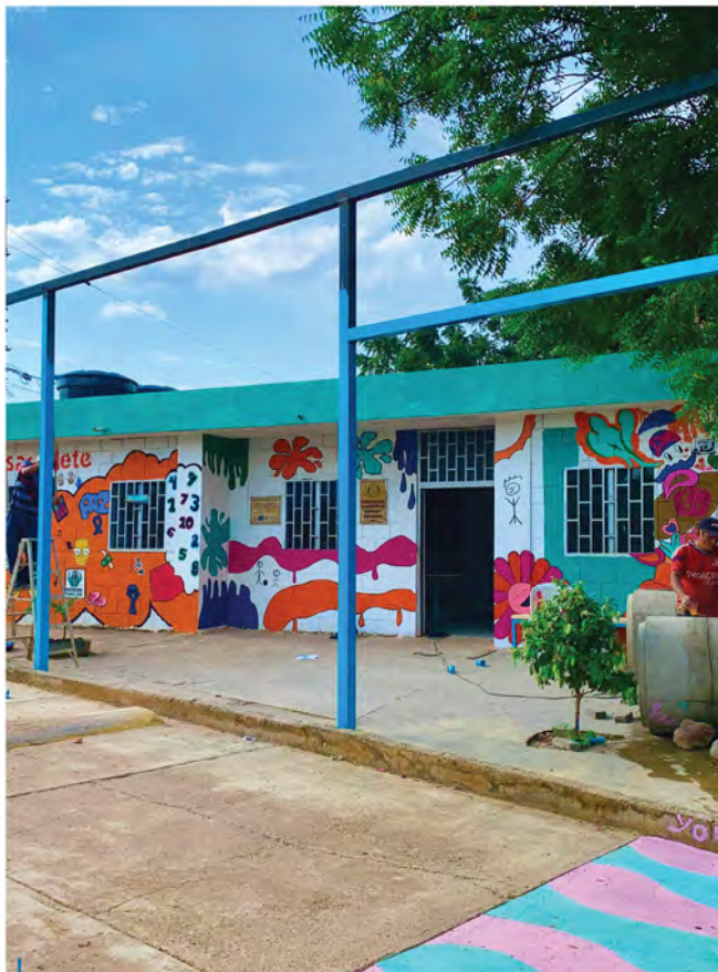
The Manuela Beltrán Community Center in Cúcuta has been restored and now functions as an inclusive public space.
