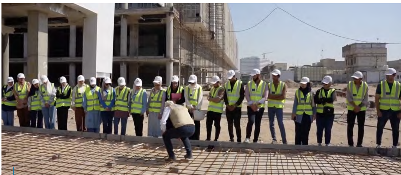
Youth participants receiving on-site training in construction techniques as part of the BEIT project.
