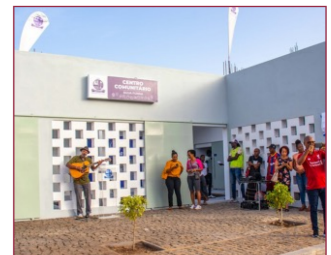
Image 61. Água Funda Community Centre in Cabo Verde. © UN-Habitat
