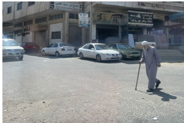
Fig. 101: Example of a main street that lacks efficient walkability infrastructure in Sahab
