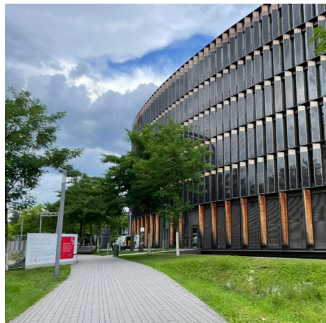
Fig. 141: The new town hall in Freiburg showing the use of PV Cells.
