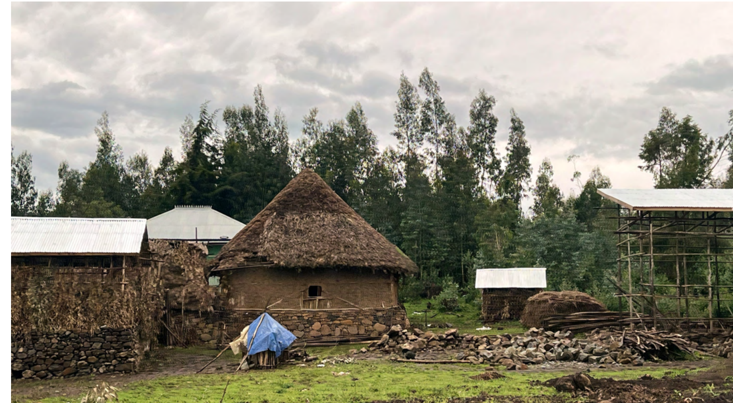
In the Chacha informal settlement of Debre Birhan, flood-affected homes reflect the compounded vulnerabilities of informal construction, limited drainage, and increasing climate-related rainfall extremes. © UN-Habitat / Lucia Gasser Hidalgo.
