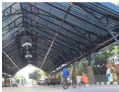
Steel shading, Bragado, Spain.
