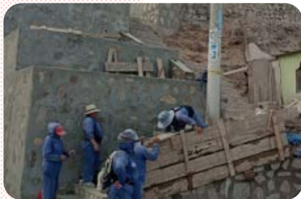
Female builders' construction work during the project © UN-Habitat
