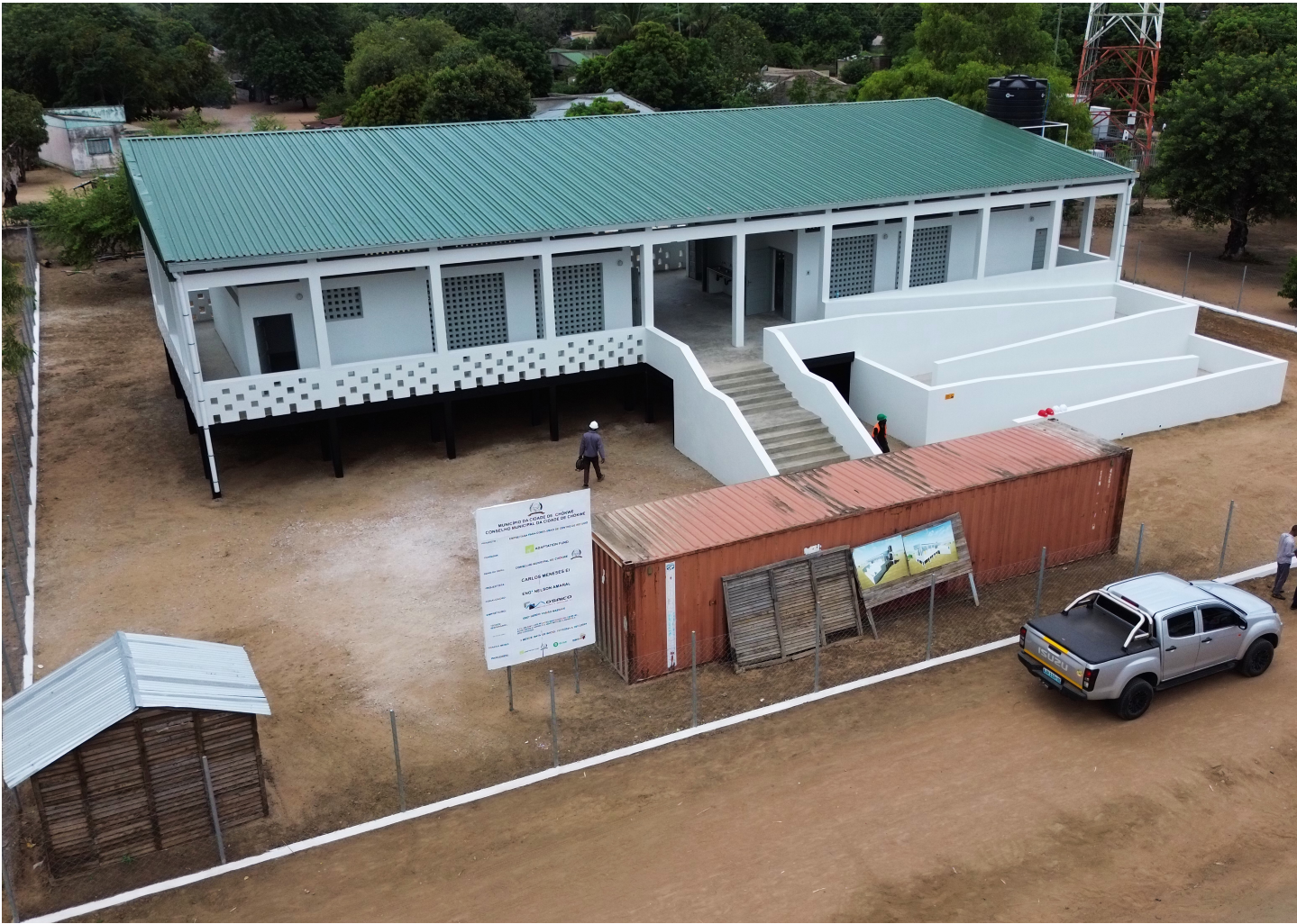
Figure 14. A multifunctional refuge centre resilient to extreme weather events in the Chókwè district, Gaza province, Mozambique. The infrastructure – built as part of a project implemented by UN-Habitat, run by Oxfam, and financed by the Adaptation Fund – provides a safe haven for the most vulnerable families in climate emergency situations, mitigating the impacts of the floods that frequently hit the region. UN-Habitat Mozambique.
