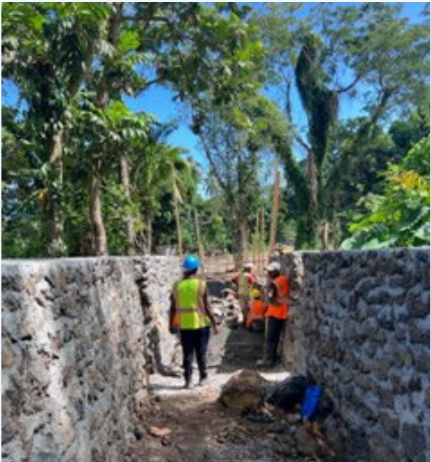
Figure 12. Drainage system construction in Moroni
