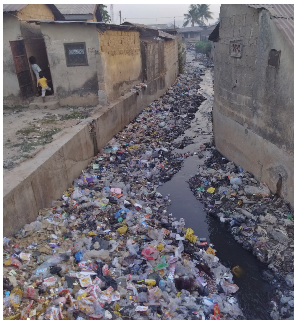
» Blocked drainage in Suleja
