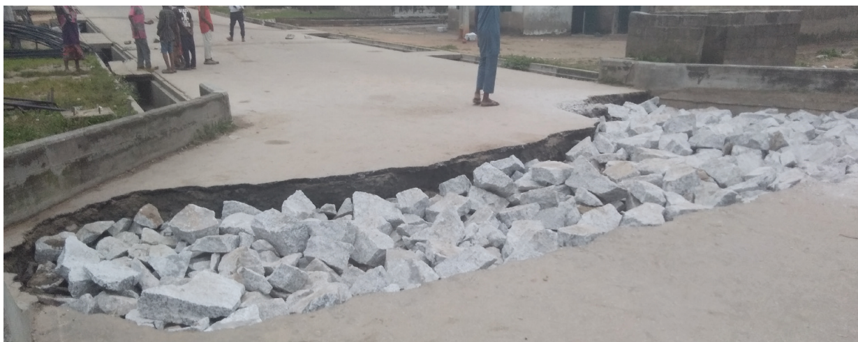
» Collapsed Okada Road as a result of flooding (Minna)
