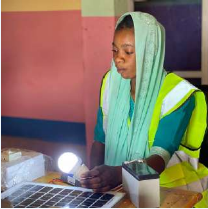
Confirmation of photovoltaic solar system functionality © UN-Habitat Cameroon
