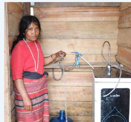
A newly built toilet with water connection to the toilet in Daksa Village in the Sekong Province © UN-Habitat Lao
