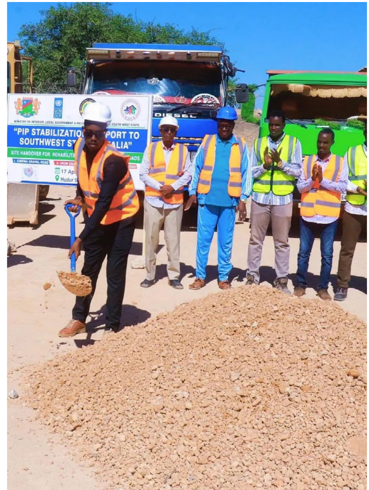
Figure 31: Road construction in Xudur with UNDP support. © UNDP Somalia, 2024
