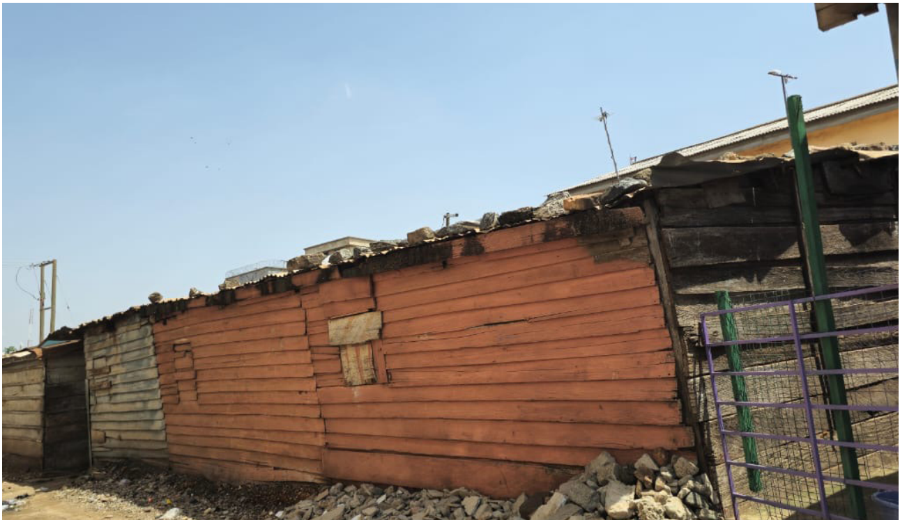
Plate 3.2: An informal housing unit built with metal sheets and wood, Accra
