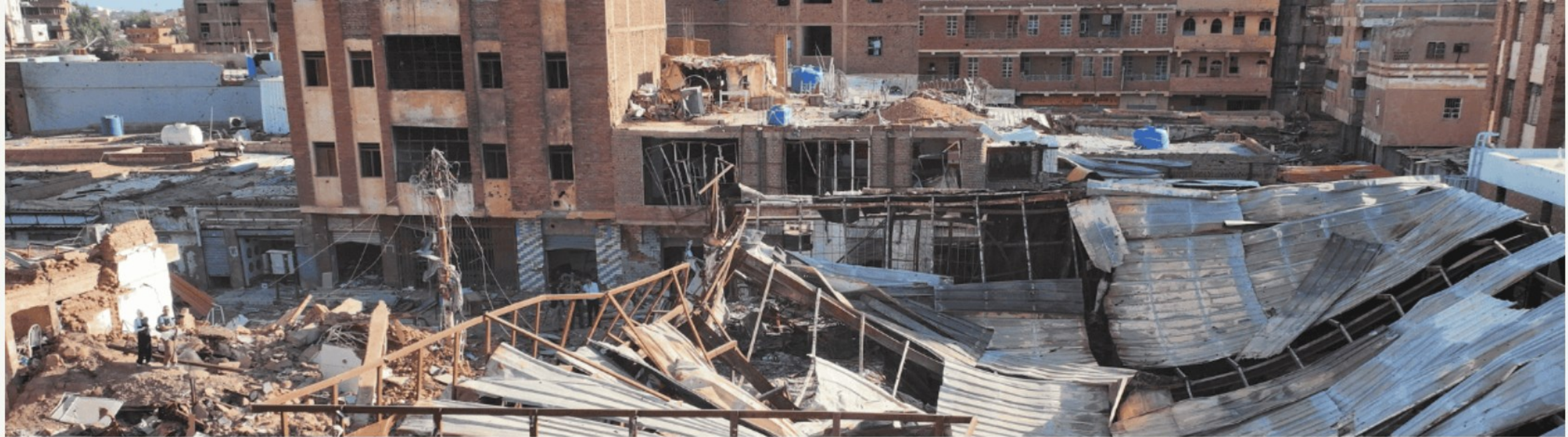
Destruction of Housing Units in Khartoum, 2024Osman Bakir / ANADOLU / Anadolu via AFP
