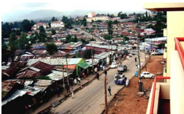
A street without storm drainage lines or sidewalks in inner Addis Ababa. Photo: © AAGG
