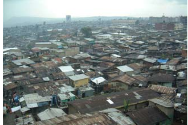
Densely built, substandard dwellings characterize most of the old residential areas of Addis Ababa. Photo: © AAGG
