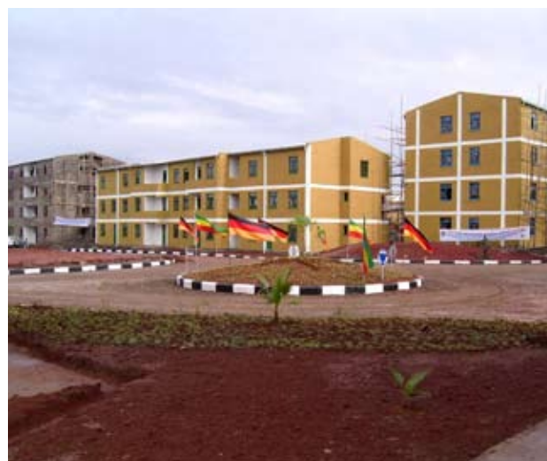
Condominium units built in the Gerji area of eastern Addis Ababa. Photo: © AAGG
