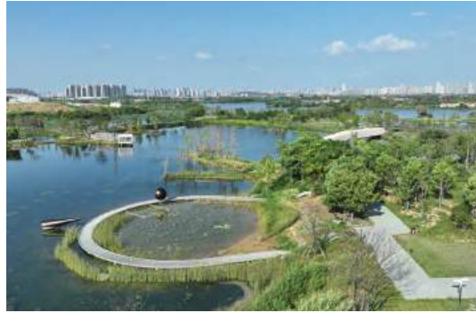
Figure 52: Bird's View of Sino-French Peninsula Town After Renovation
