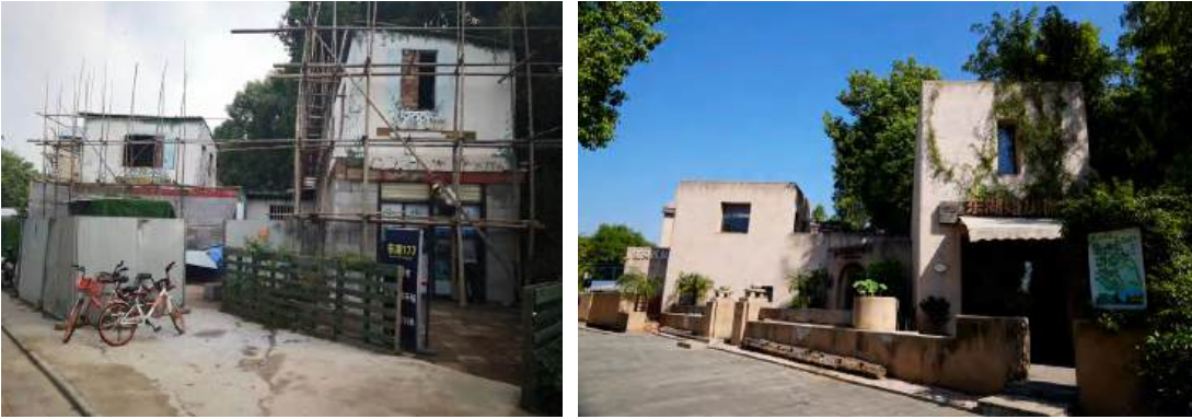
Figure 52: Pompei Restaurant Before and After the Renovation
