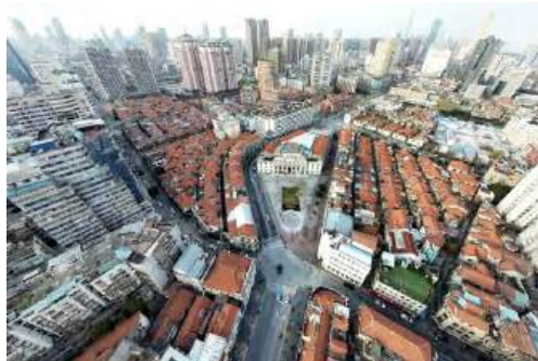
Figure 4: Renovation of Zhongshan Avenue, Wuhan
