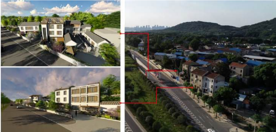
Figure 56: Buildings After (Left) the Renovation and Status Quo (Right)
