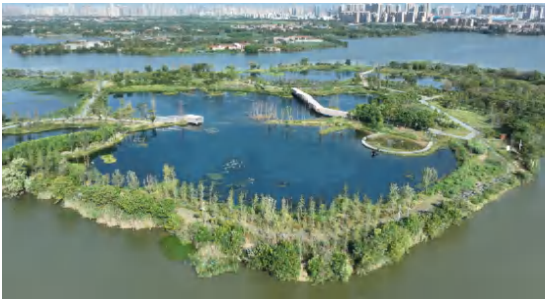
Figure80: Photo of Sino-French Peninsula Town After Renovation
