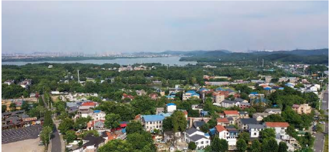
Figure 57: East Lake Dali Village After the Small-scale Renovation
