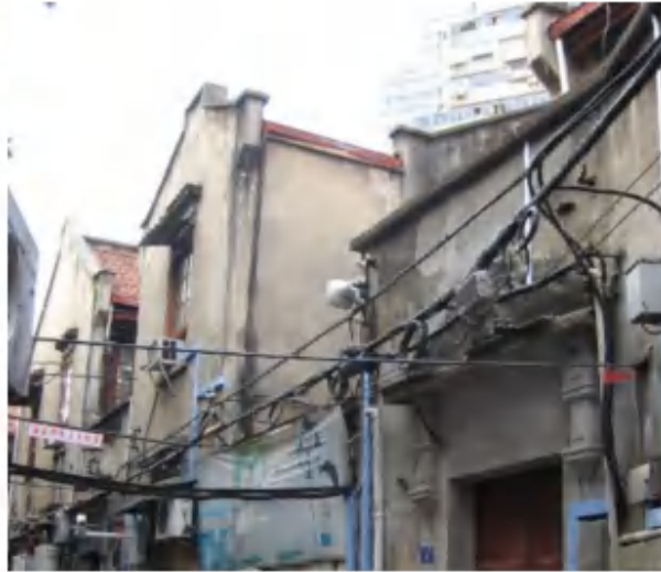
Figure 90: Cornice Parapet of Baoyuanli Before the Renovation
