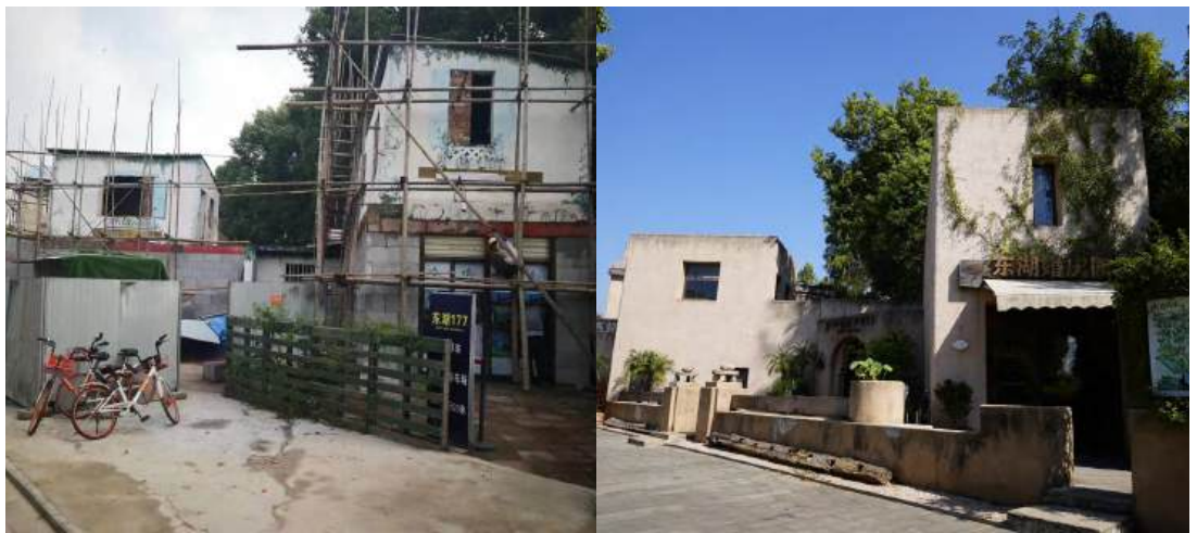
Figure 43 : Pompei Restaurant Before and After Renovation
