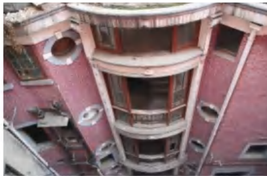
Figure 88: Internal Facade of Jinchengli Before the Renovation
