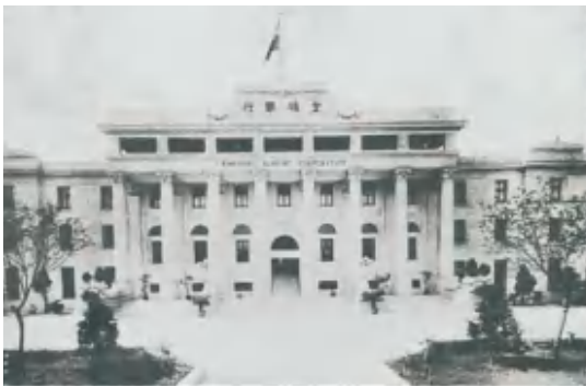
Figure 87: Historical Photo of Jincheng Bank
