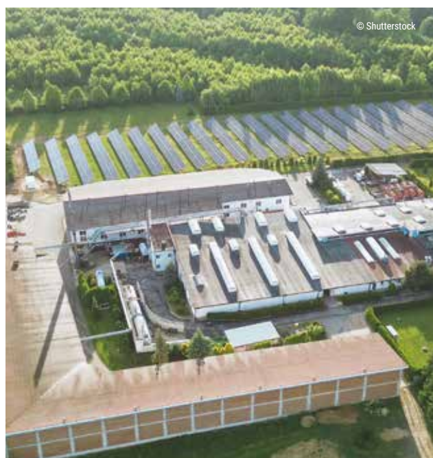
Sustainable Industrial Facility with Solar Power Plant
