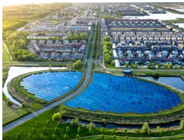
Sustainable neighbourhood in Almere, The Netherlands. The city heating (stadswarmte) in the district is partially powered by a solar panel island (Zoneiland) © Shutterstock
