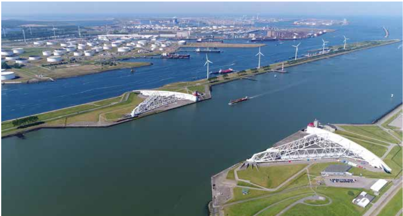
Storm surge barrier, Rotterdam, Netherlands © Shutterstock
