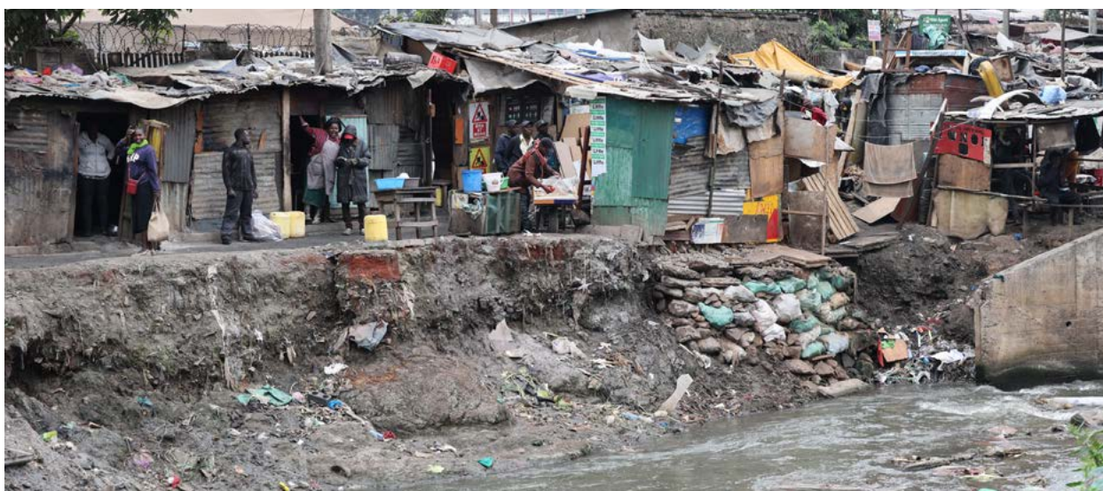
FIGURE 8 Flood-prone informal settlements in Nairobi, Kenya Source: © UN-Habitat_Julius Mwelu, 2024
