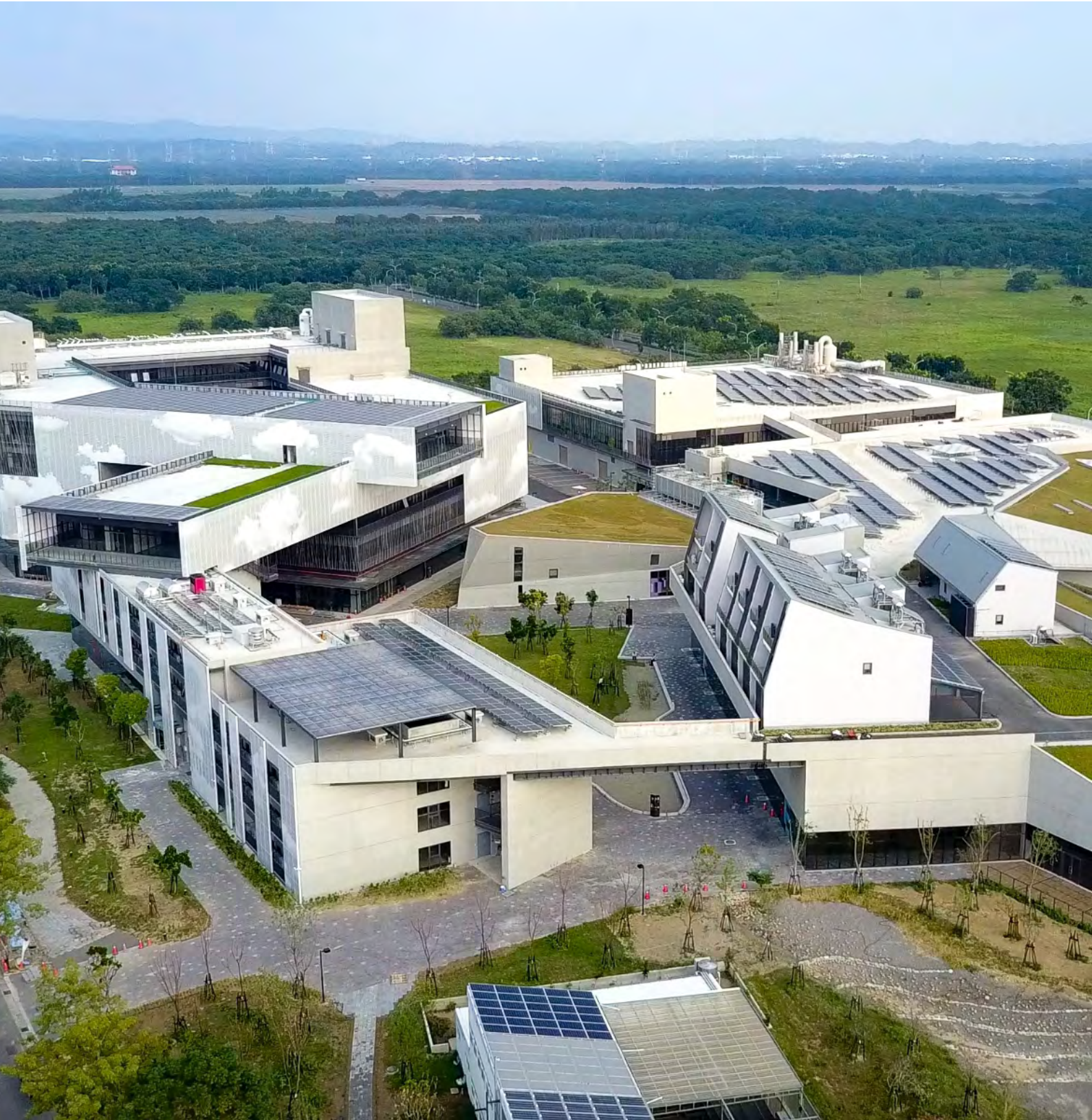
△ Shalun Smart Green Energy Science City
