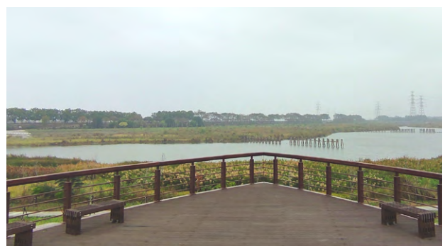
△ Tainan's Largest Flood Storage Pond - Su Chu Flood Storage Pond
