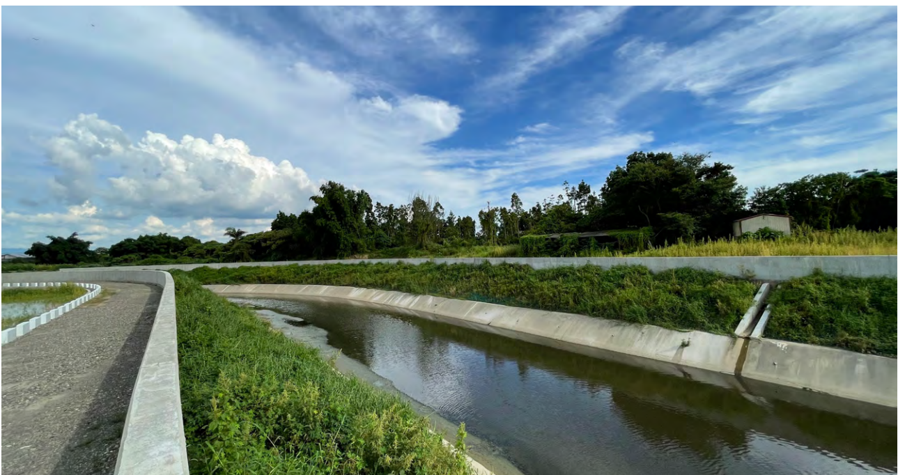
△Gueizi Harbor Drainage Shoreline Treatment Project (3K+943~4K+241)
