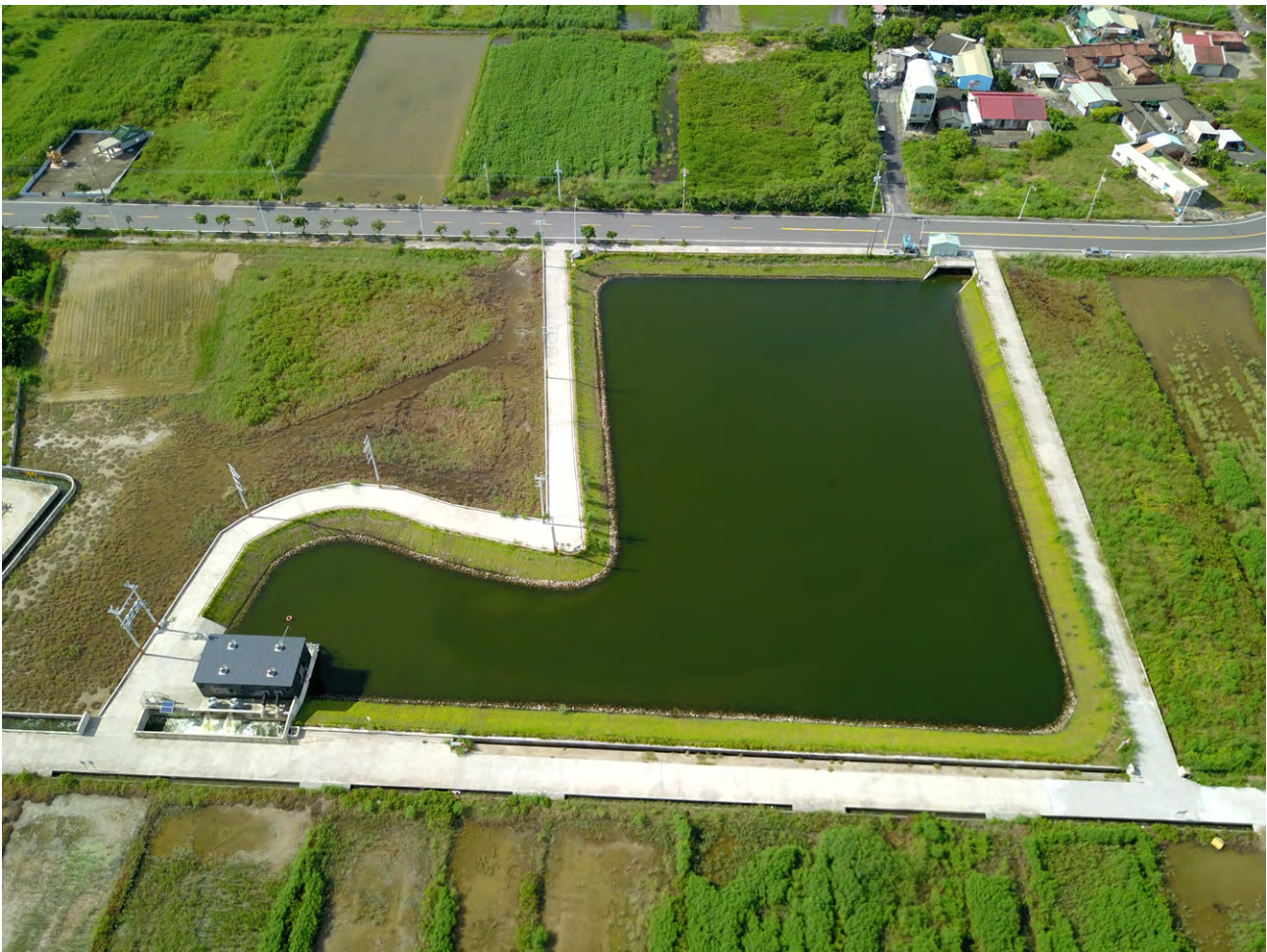
△ The General Guangshan Flood Storage Pond, with the Appearance of a Giant Christmas Boot
