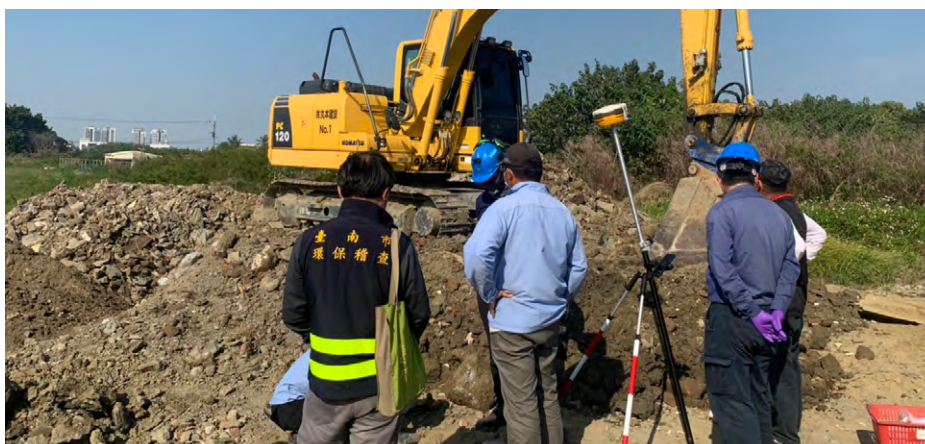
△ Supervision of Site Pollution Remediation
