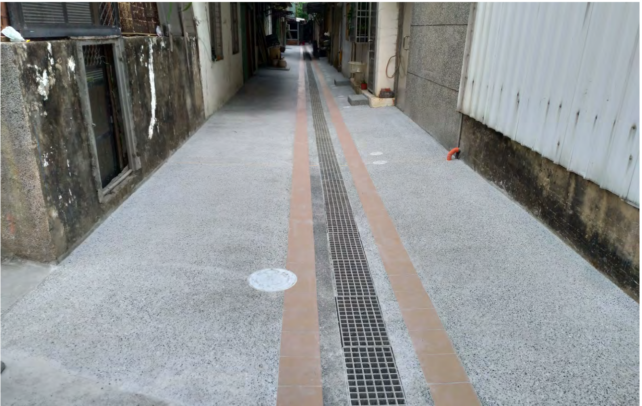
△ Waste Water Sewer
