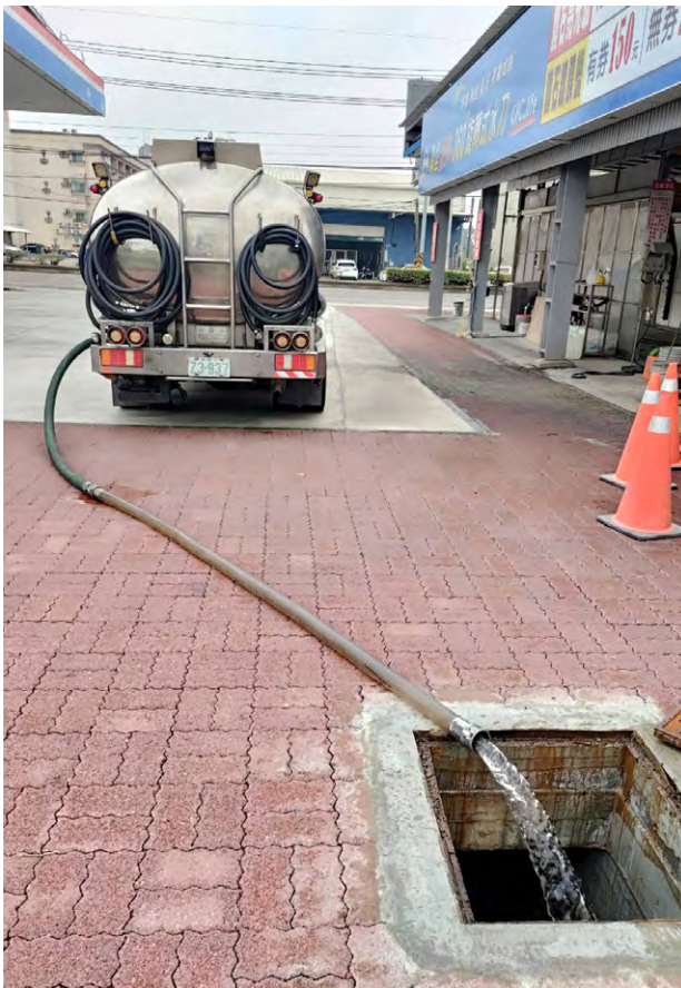
△ Water Tankers Dispatched in Emergency to Support Gas Stations
