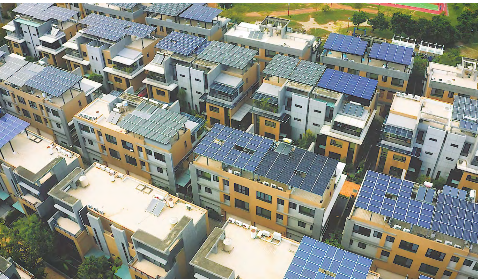
△ Green Roofing in Tainan City's Annan District
