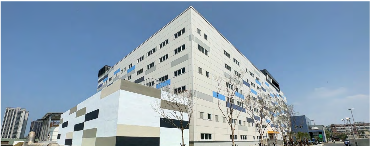
△Anping Water Reclamation Plant
