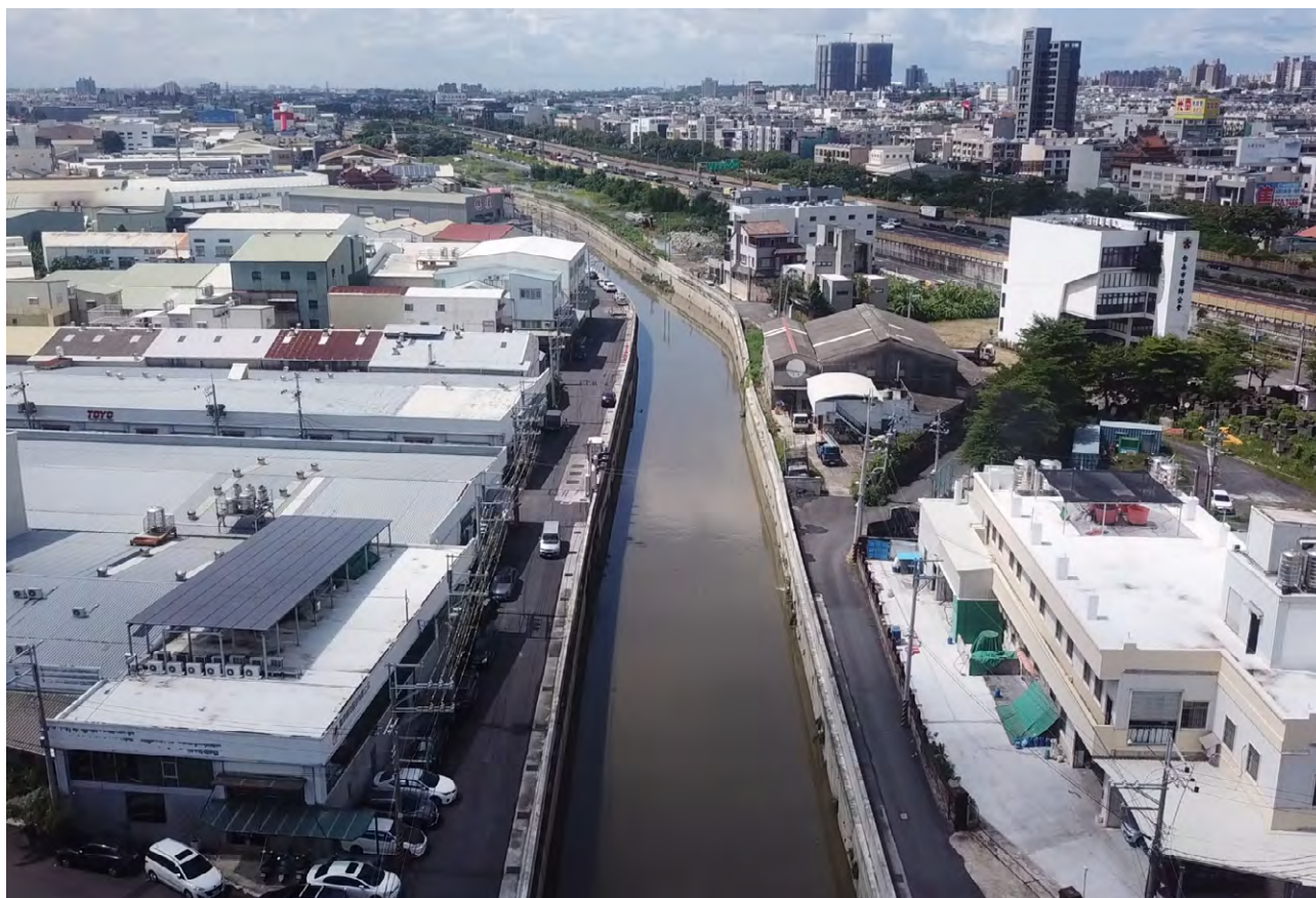
△ Remediation of the Upper Sanyi Creek has been completed
