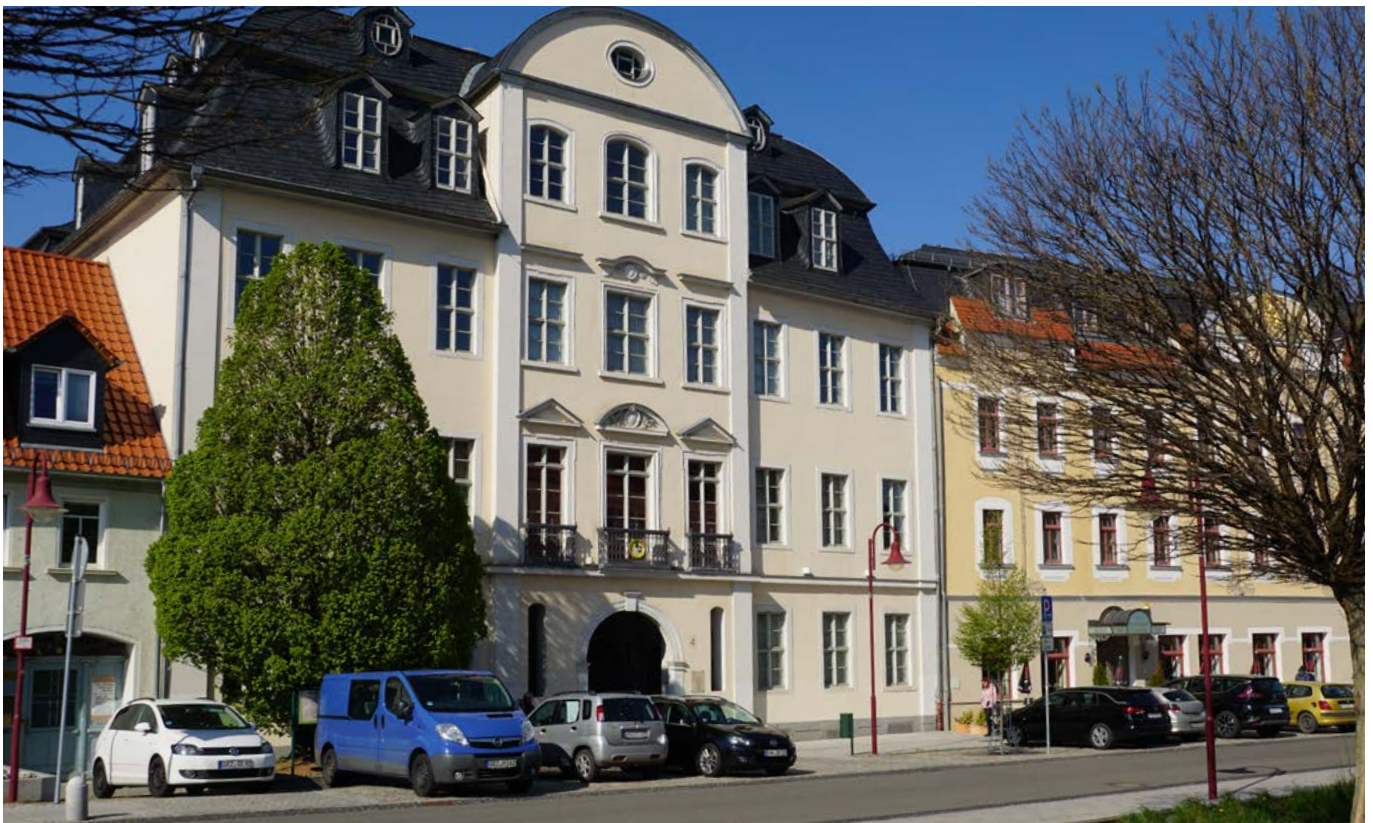
Photo 14: Establishment of a public toilet in the city hall (palace building) © Stadt Bad Köstritz
