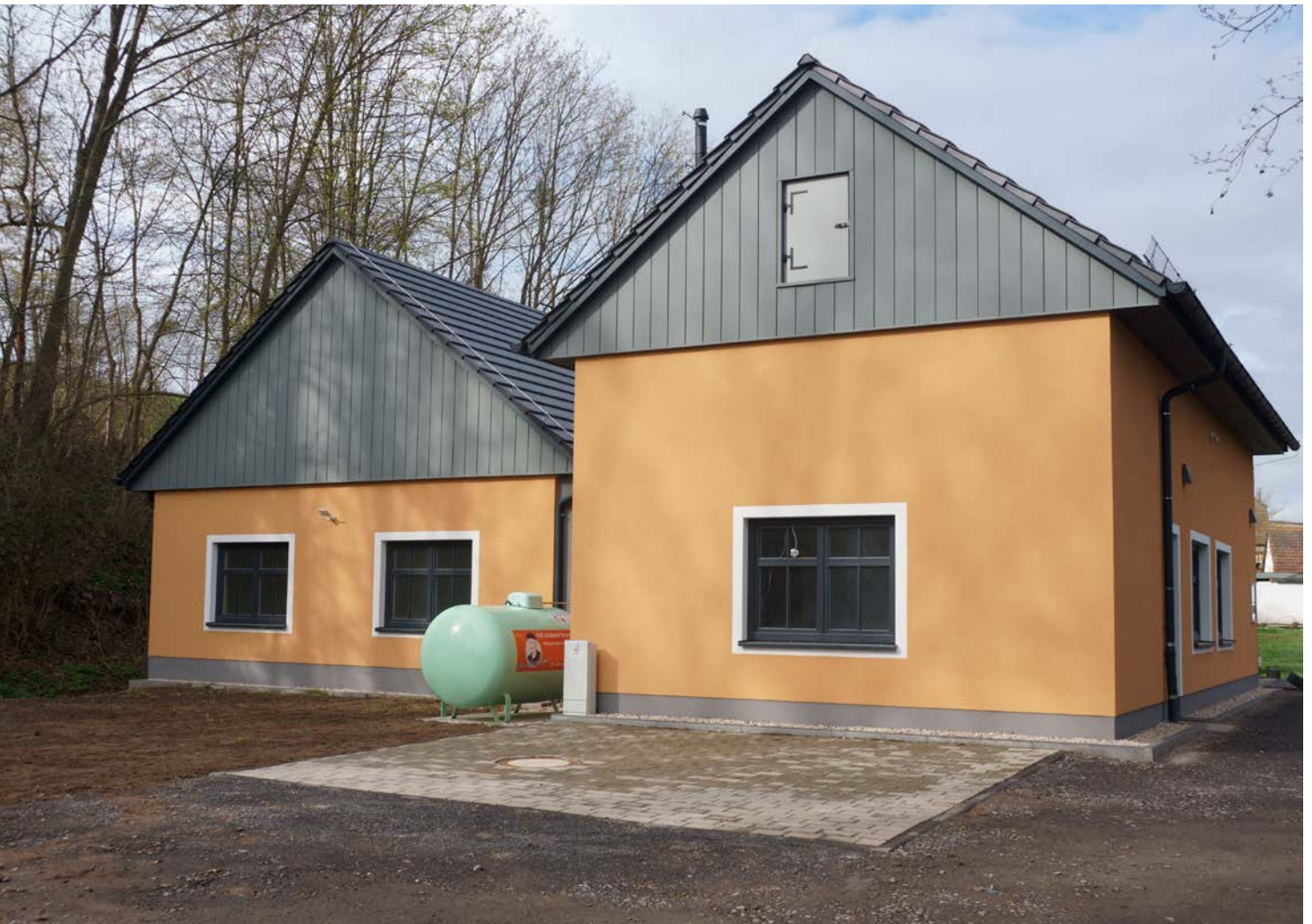
Photo 11: Village community center in the district of Reichardttsdorf with biological sewage treatment plant © Stadt Bad Köstritz
