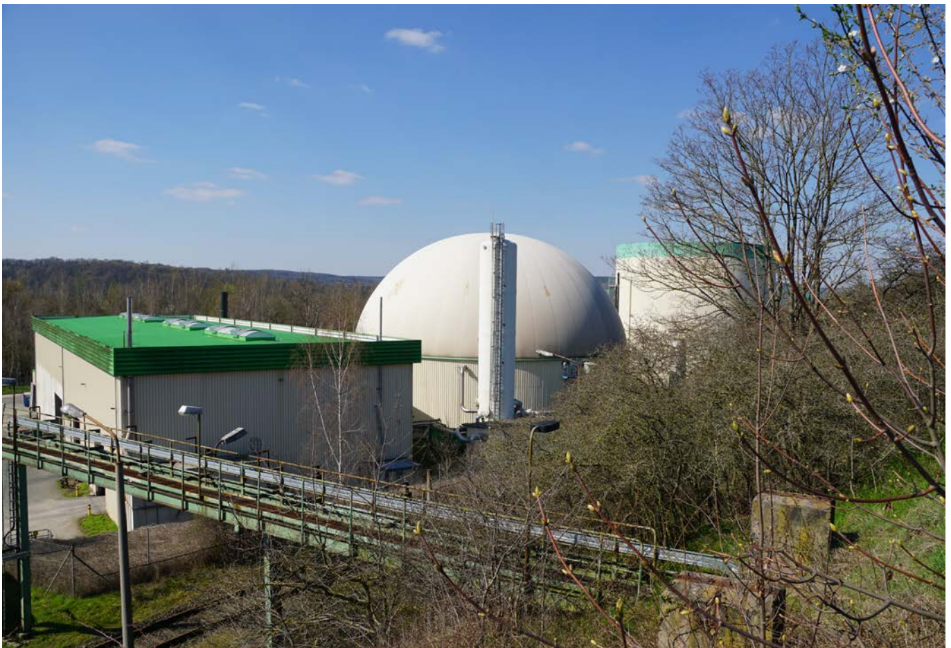
Photo 17: Bioenergy plant © Stadt Bad Köstritz
