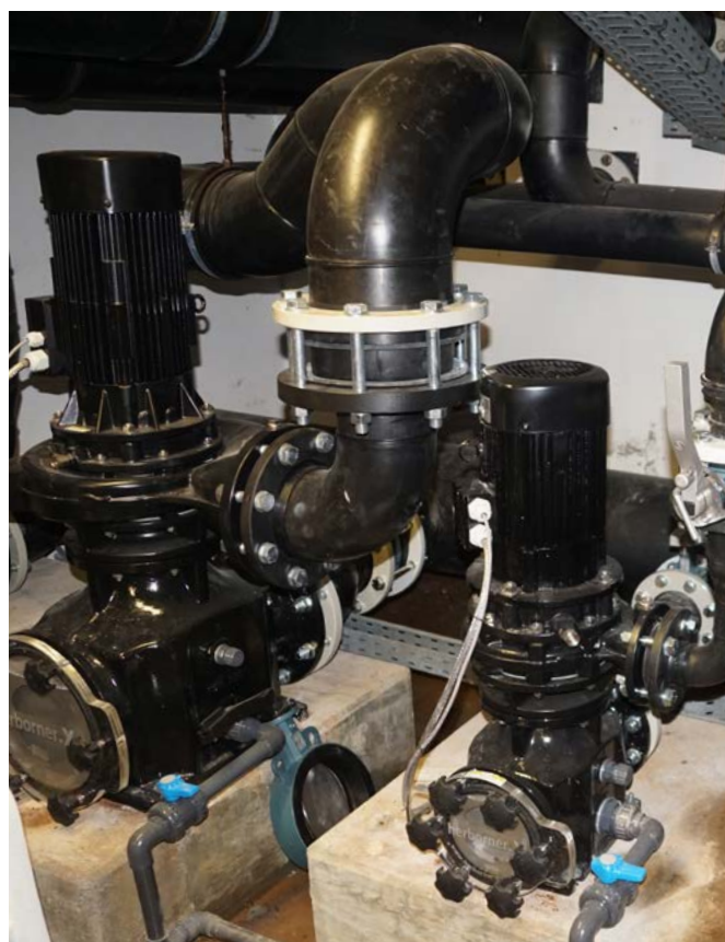
Photo 19: Renewal with energy-efficient pumps in the leisure and recreation baths © Stadt Bad Köstritz
