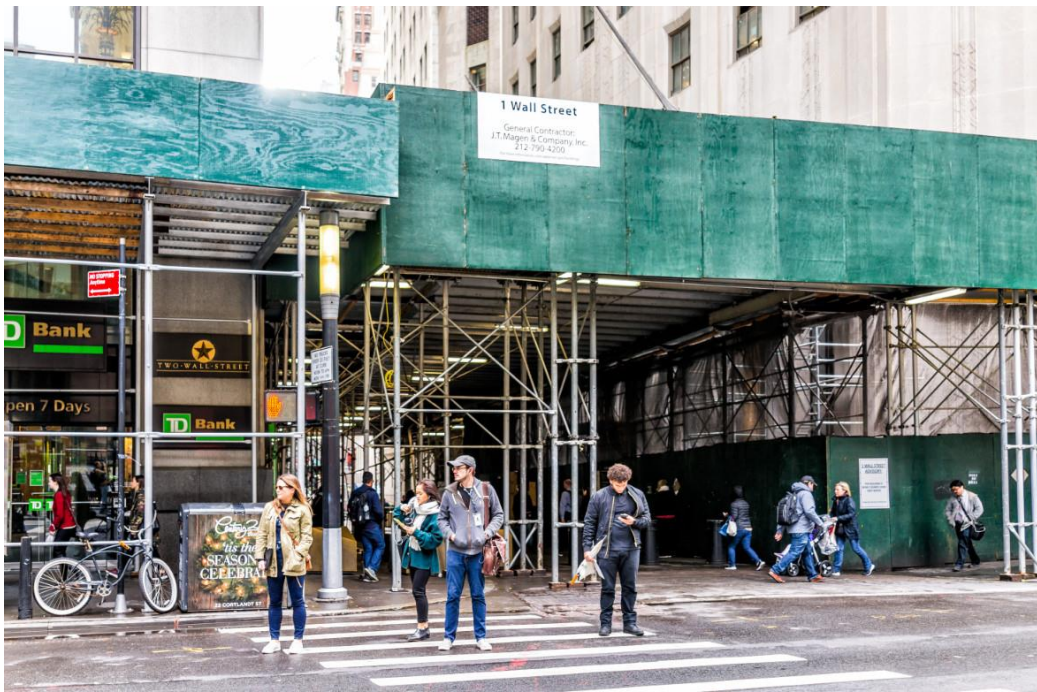
Overhead canopy with safety nets, accessible from Google Image, accessed on 10/11/23
