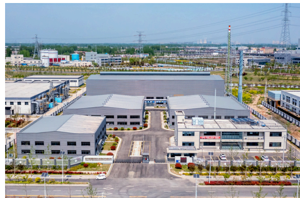
Figure 2-13 Saturated Activated Carbon Regeneration Project © Xuzhou Municipal Urban Administration Bureau
