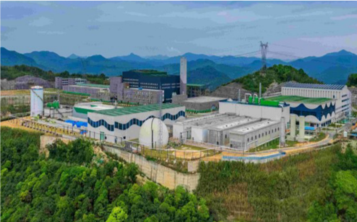
Figure 3-9 Fuzhou Food Waste Treatment Plant © Fuzhou Municipal Urban Management Committee
