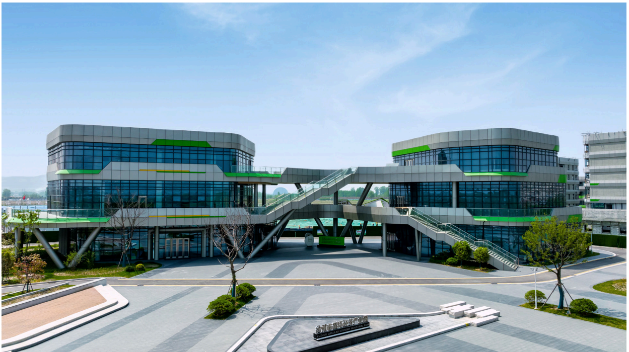
Figure 2-14 China "Zero waste City" Culture Exhibition Hall and China Circular Economy Industry Expo Hall © Xuzhou Xincheng Lvyuan Circular Economy Industry Investment and Development Co., Ltd
