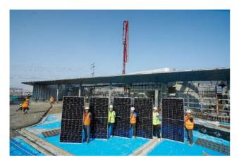
Figure 4-2: installment of photovoltaic system Source: Shanghai Zhenru
