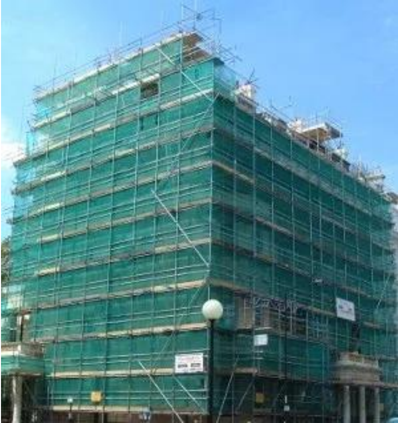
Scaffold net, accessible from Google image, accessed on 10/11/23
