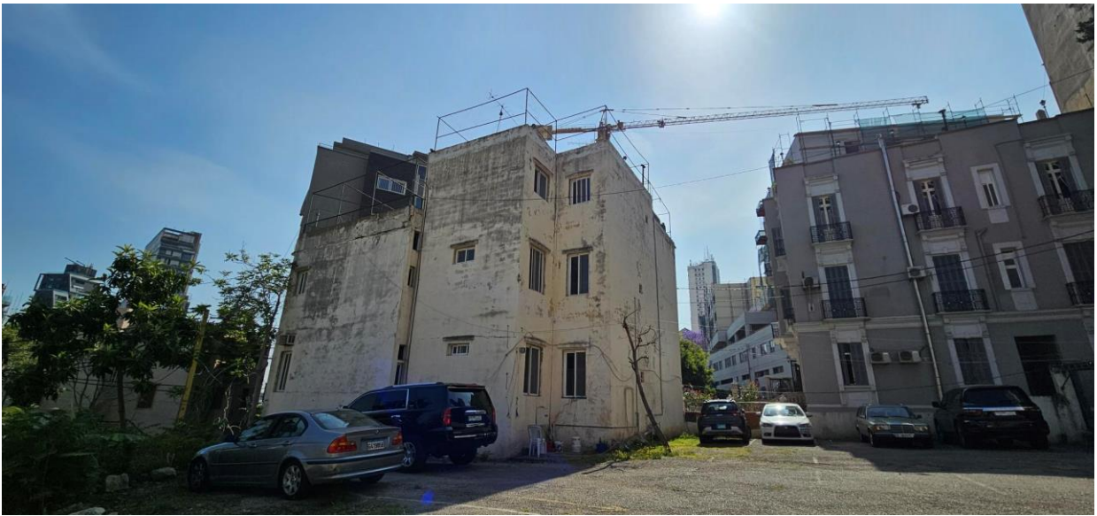
Figure 3: Picture of Re_738 façade (UN-Habitat, 2023)
