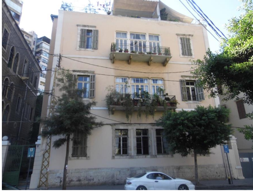
Figure 10: Re_692 main elevation before the blast (BBHR, 2020)
