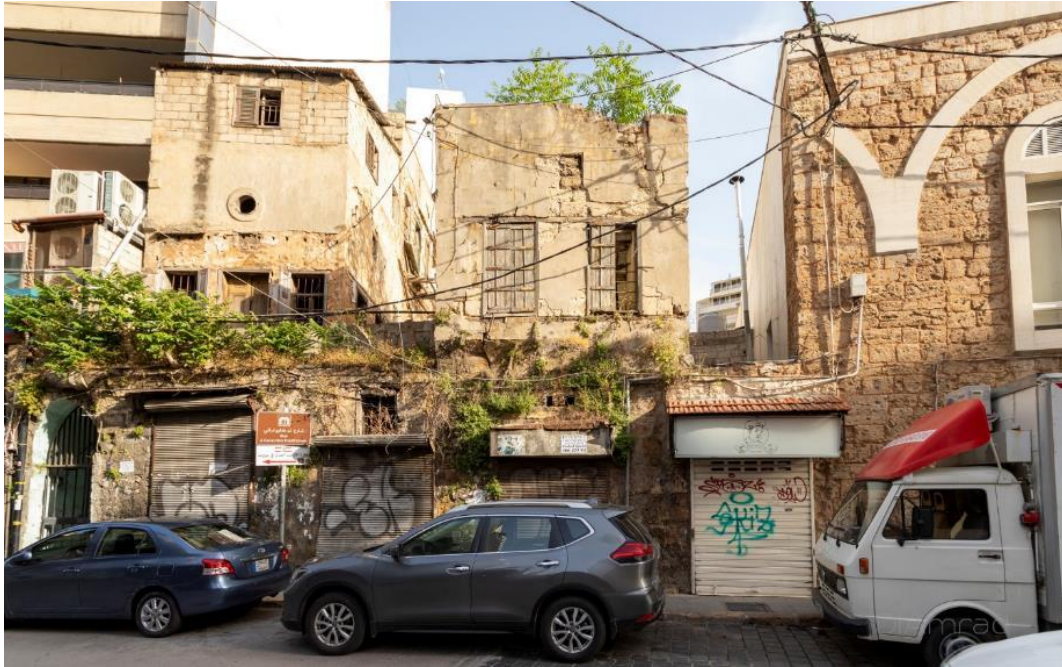
Figure 6: Re 364 before the blast (Dia Mrad 2019)
