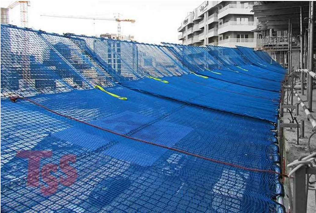
Safety nets, accessible from: tss-me.com/blog-posts/all-about-construction-safety-nets/ , accessed on 10/01/23
