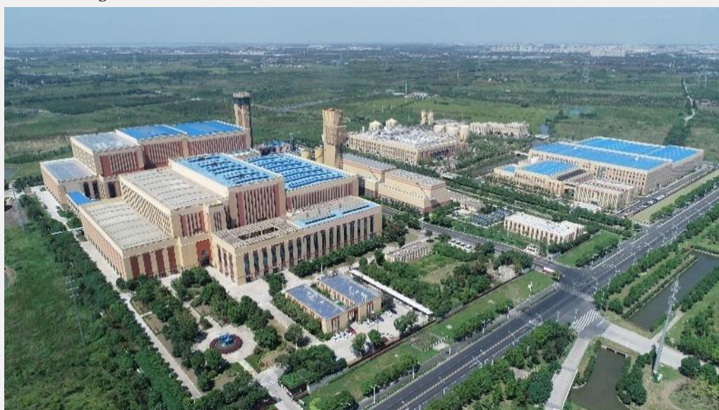
Figure 25 Incineration Plant in Tianma Zero-waste Low-carbon Eco-friendly Industrial Park in Songjiang District
