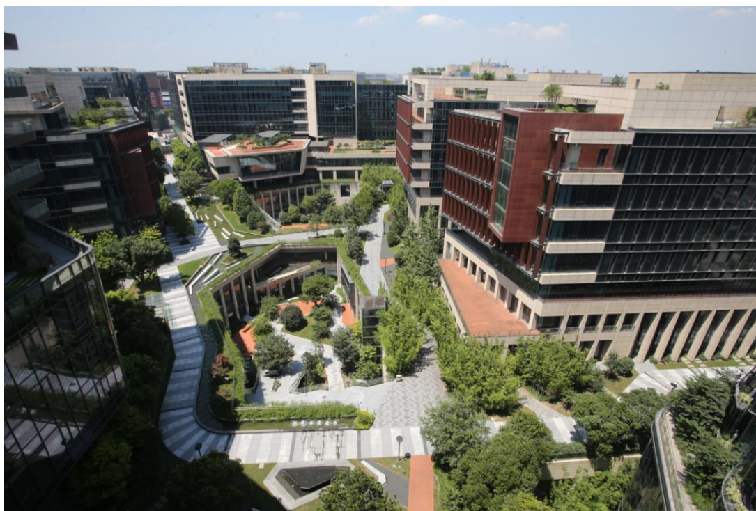
Figure 26 Hongqiao Green Valley Plaza
