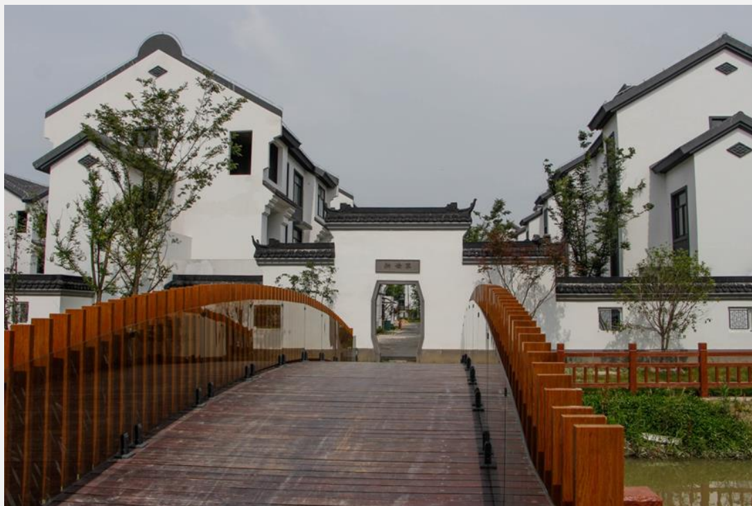
Figure 15 Village Appearance after Rectification
