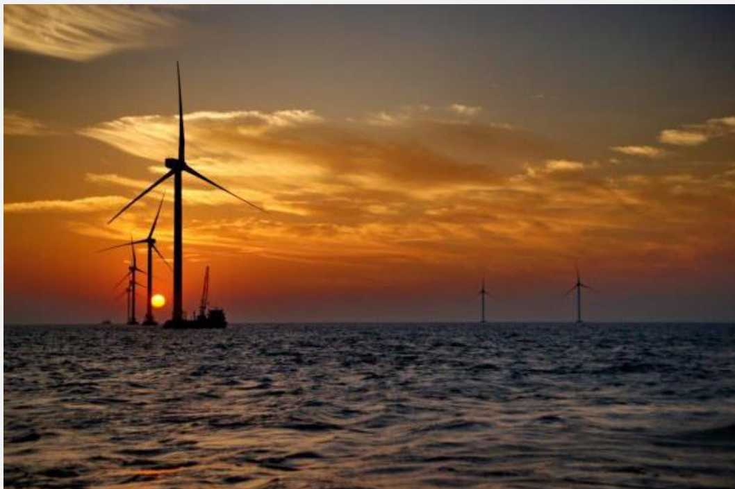
Figure 10 Offshore Wind Farm near Donghai Bridge, Shanghai
