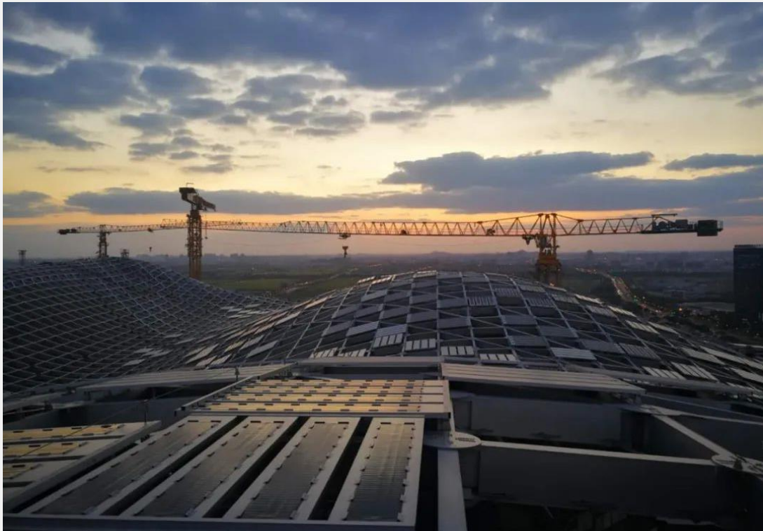
Figure 11 Rooftop of G60 S&T Innovation Valley
