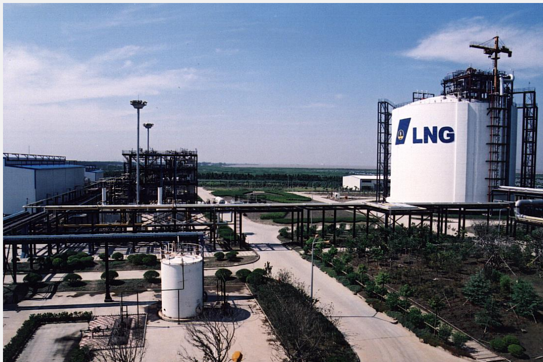
Figure 11 LNG Terminal in Wuhaogou, Pudong New Area
