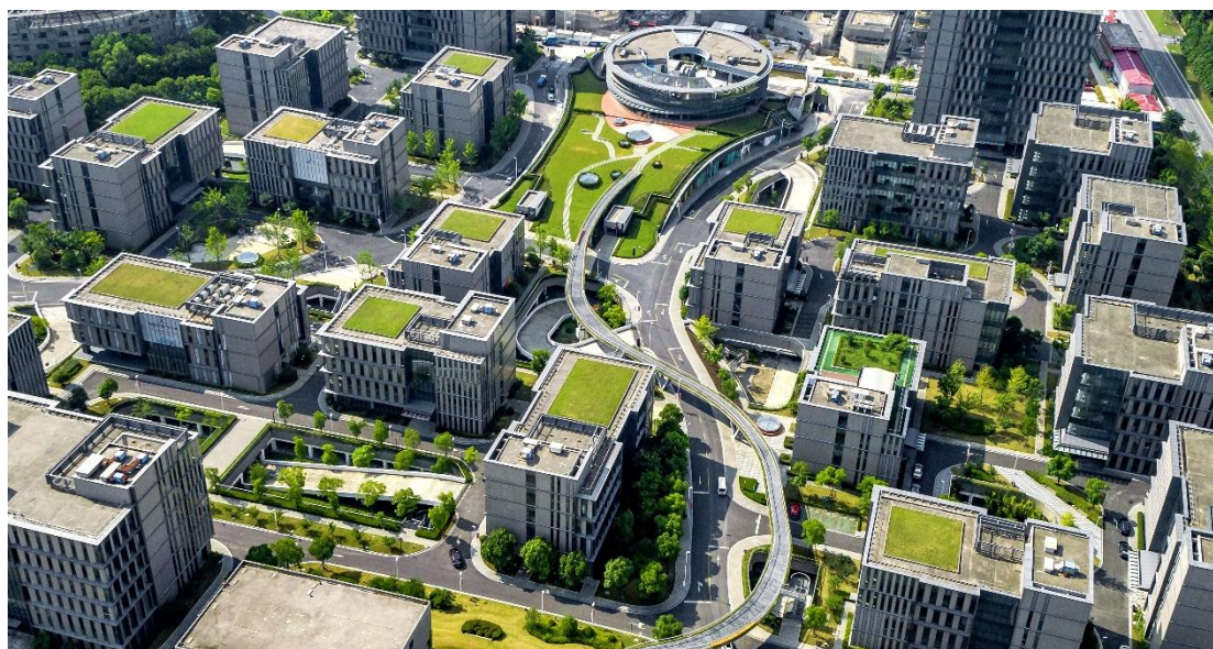
Figure 23 Lingang Nanqiao Science and Technology Park
