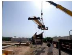
Delivery of 2 bridge cranes for pumping station
