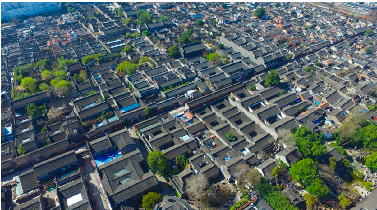
Figure 5-2 Aerial View of Dongguan Street
