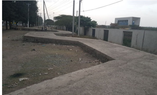
Construction of foundation for partially relocated market in Hawassa
