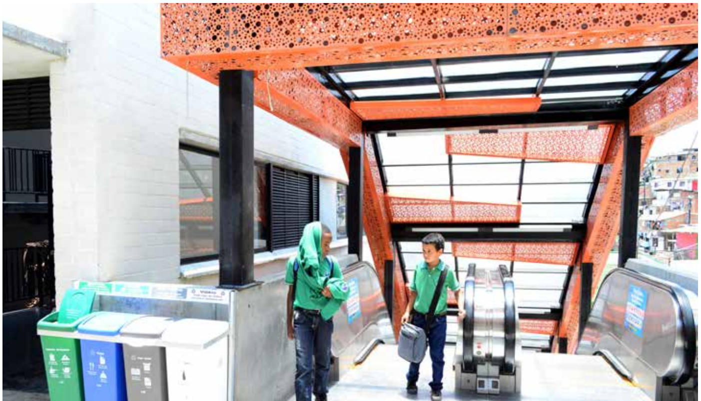
Children come up the escalators in '20 de Julio' neighborhood in Comuna 13 slums in Medellín, Colombia © Julius Mwelu/UN-Habitat
