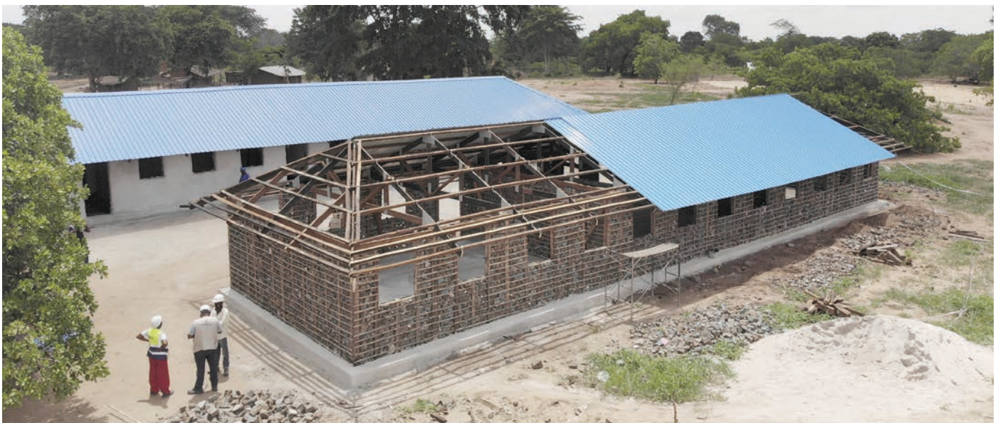
Building mixed material resilient schools in Nampula, Mozambique © UN-Habitat
