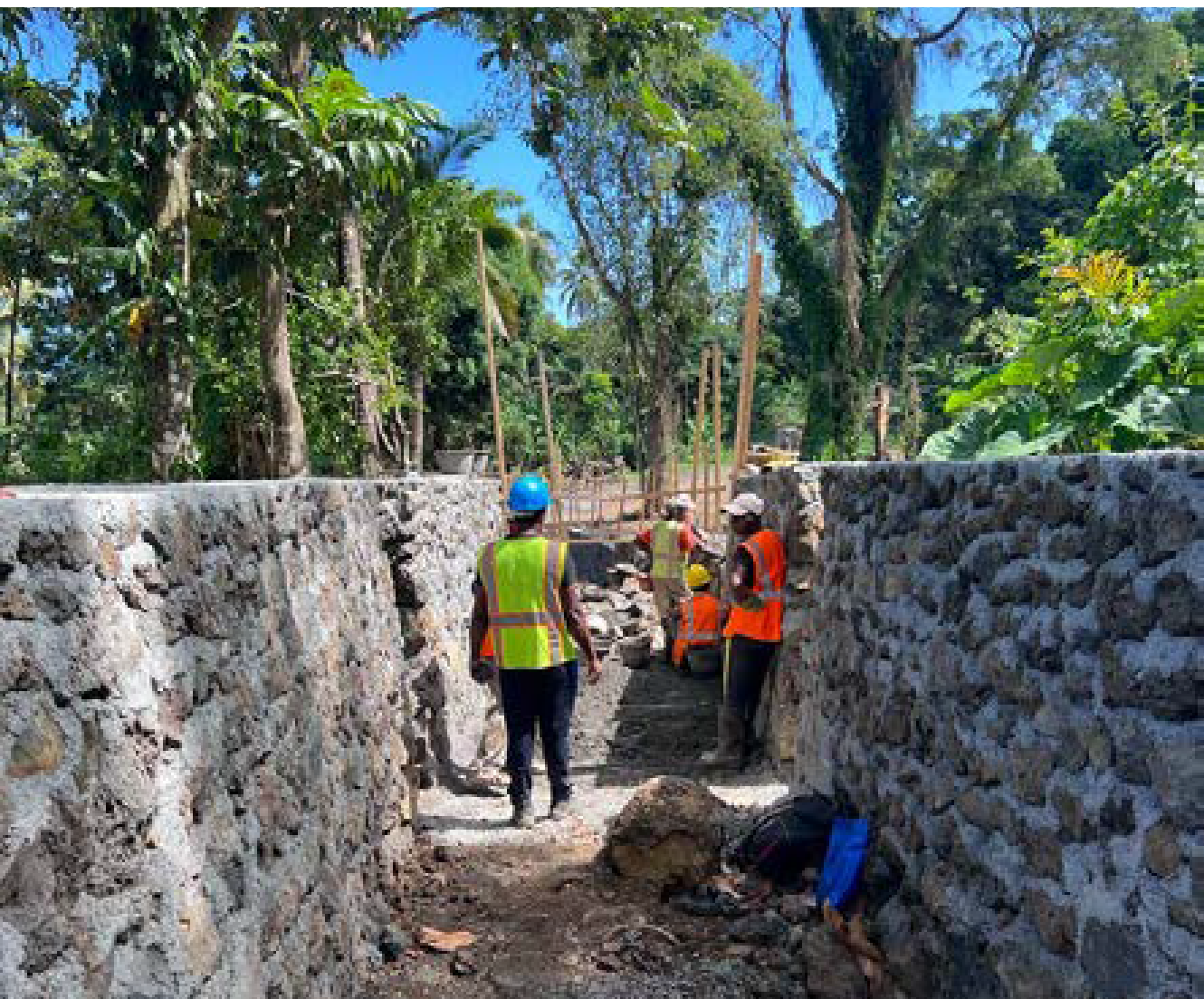
Drainage capacity development in La Coulée; work in progress. Credit: OXFAM
