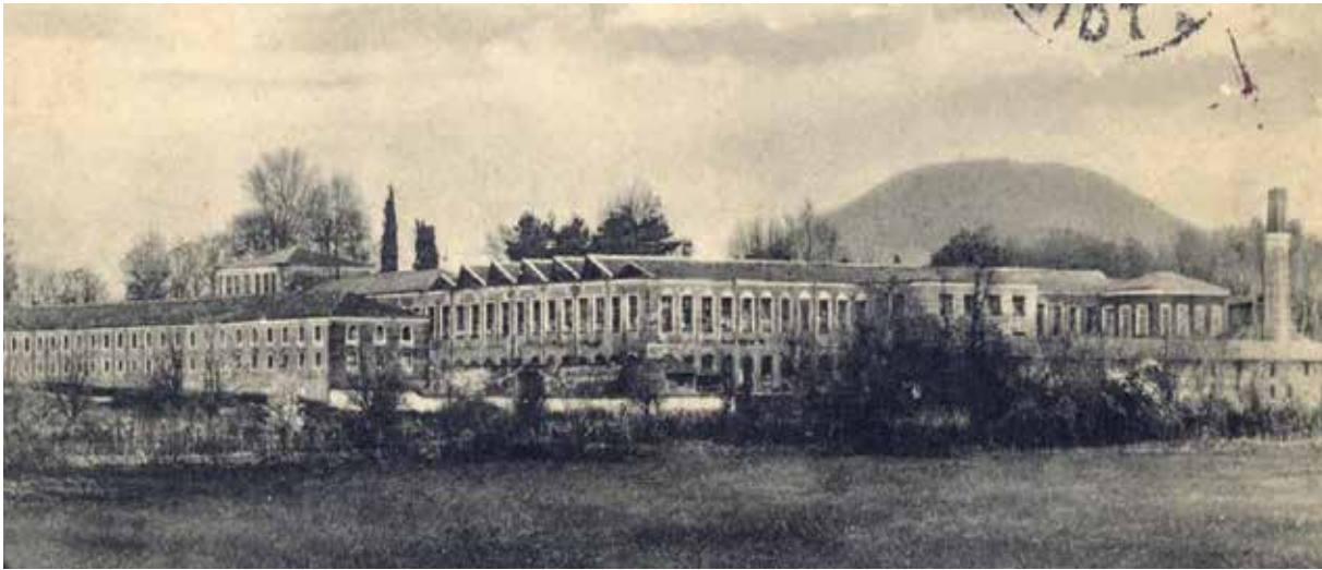
View of the Çuha Factory in Early 20th Century
