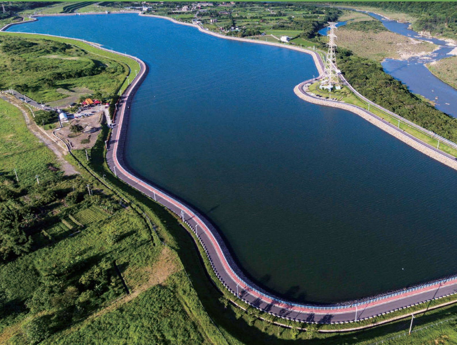
Daxi Zhongzhuang Adjustment Pool and Peripheral Trails / Credit: Northern Region Water Resources Office, Water Resources Agency, Ministry of Economic Affairs
