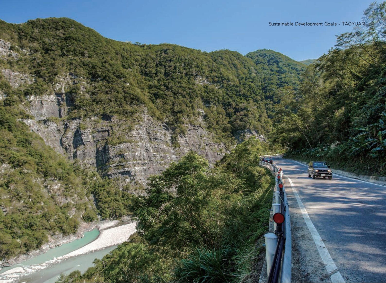
North Cross-Island Highway Section in Fuxing Dist.
