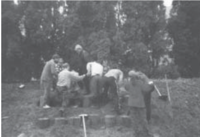
The playground construction begins through volunteer work!
