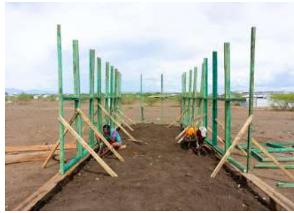
Right: Type E Pilot Shelter Construction - Frame Construction Process. © UN-Habitat
