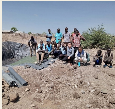
Construction team including Daiken and local masons. © UN-Habitat
