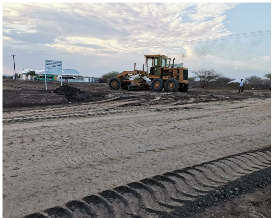
STEIN chemical spread across the road, awaiting compaction. © UN-Habitat
