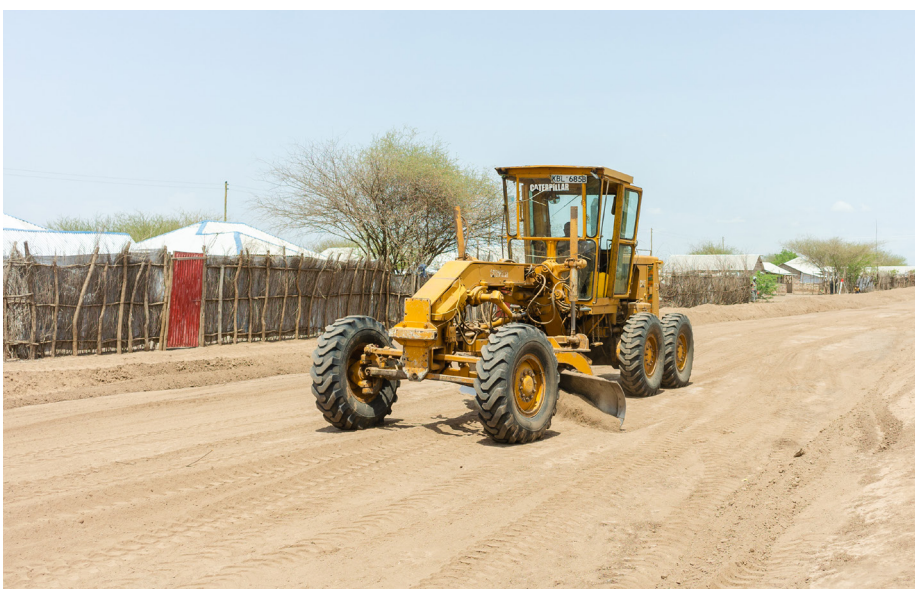
A grader carrying out the initial road earthwork. © UN-Habitat
