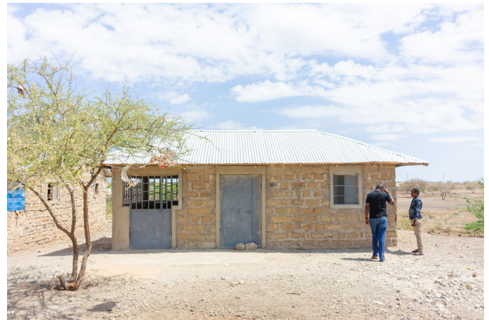
UN-Habitat Team checking a near complete shelter. © UN-Habitat
