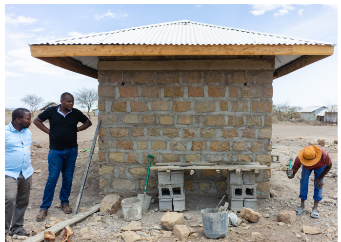
A mason finalising on shelter finishings. © UN-Habitat
