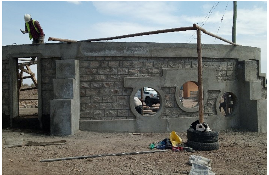
Construction of amphitheater. © UN-Habitat
