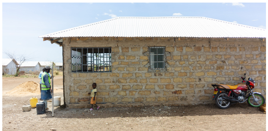
Shelter with metallic window grills. © UN-Habitat
