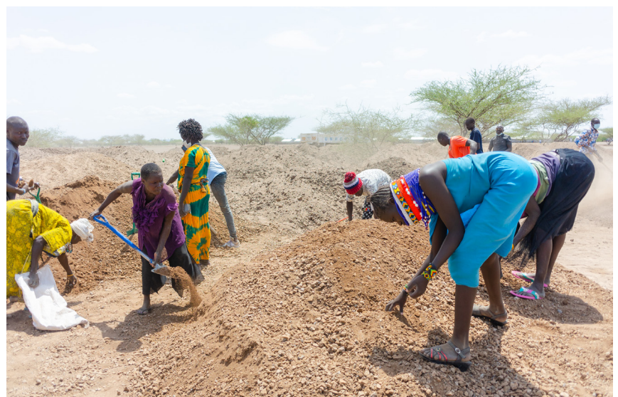
Host and Refugees carrying out soil pulverisation for STEIN Road. © UN-Habitat
