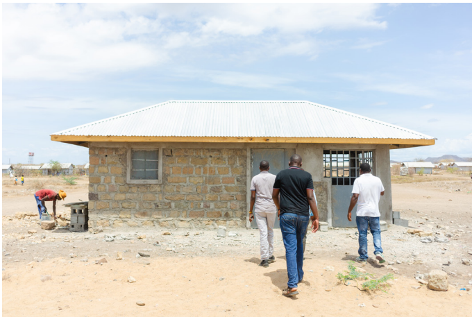
UN-Habitat and NCKK Technical team inspecting a completed shelter. © UN-Habitat
