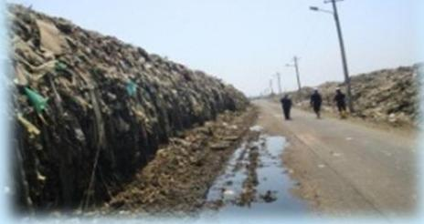
Prevented collapse by making slope milder
