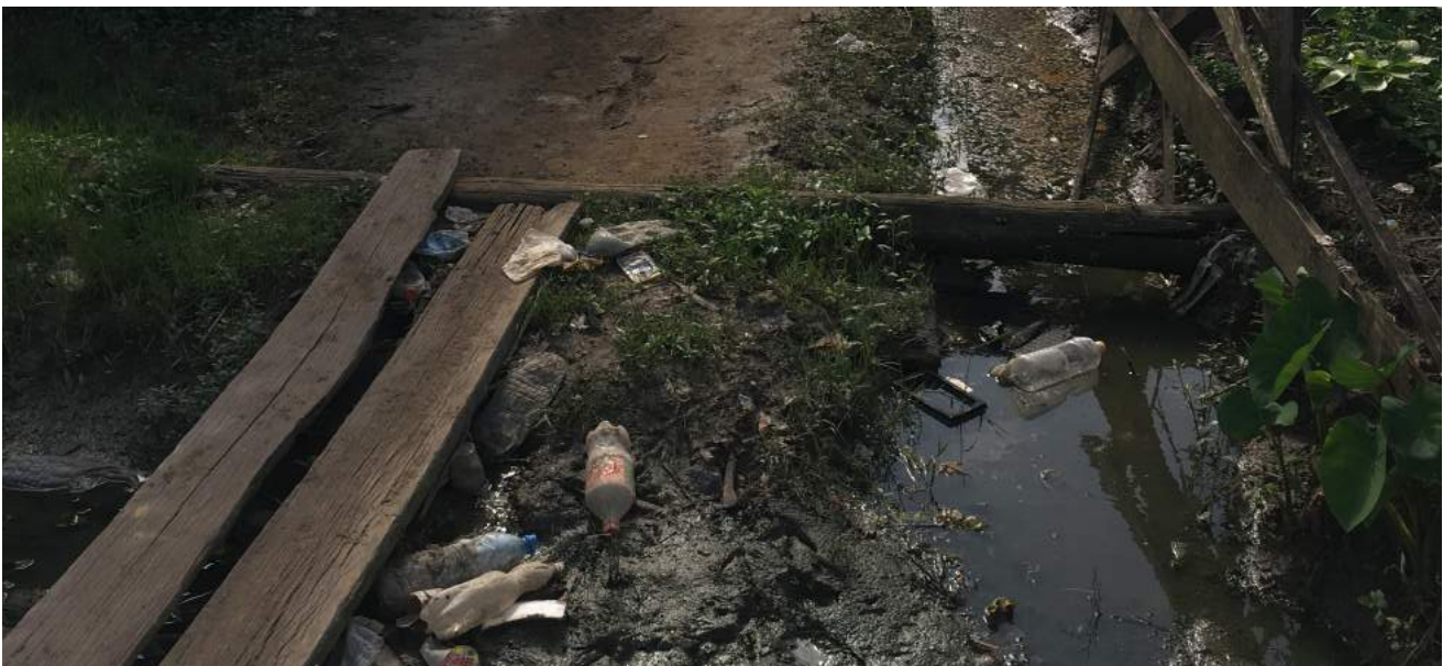
Photo 20. To cross flooded roads, wooden boards are used as makeshift mini-bridges Source: UN-Habitat
