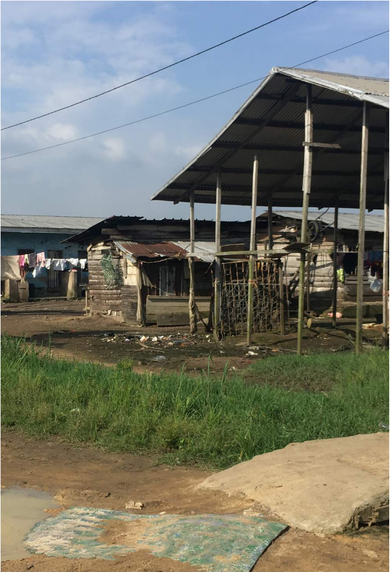
Photo 16. Wooden "case" housing accomodating IDPs near the banks of the Wouri River Source: UN-Habitat
