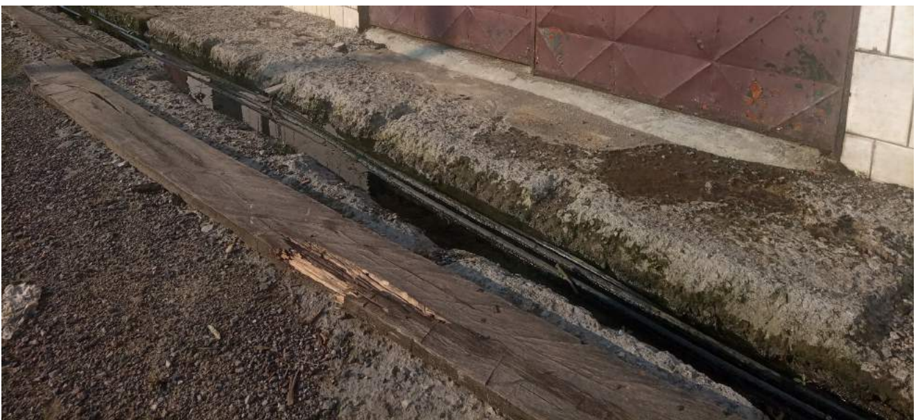
Photo 13. A rainwater drainage gutter. Source: UN-Habitat
