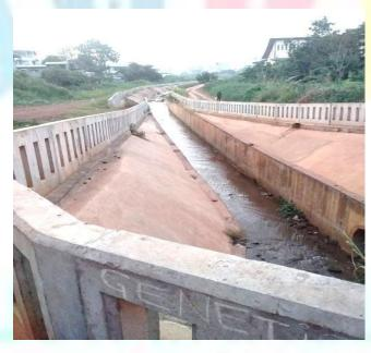
Figure 3: Arrangement of the Mfoundi bed to reduce flooding
