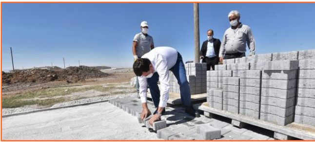
Image 52: Street paving works
