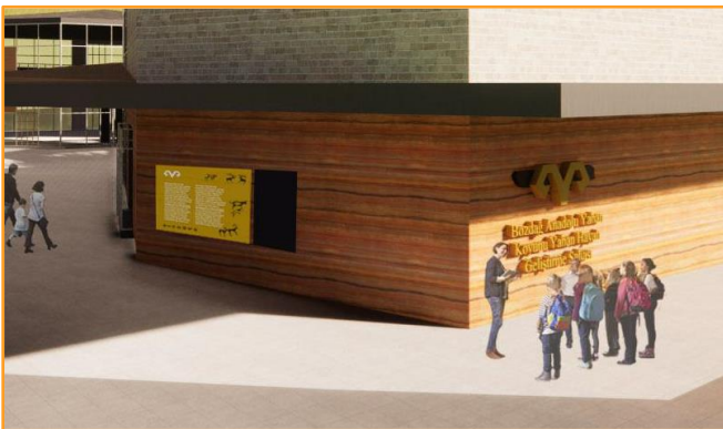
Figure 29: The use of local materials in architecture (compressed soil)
