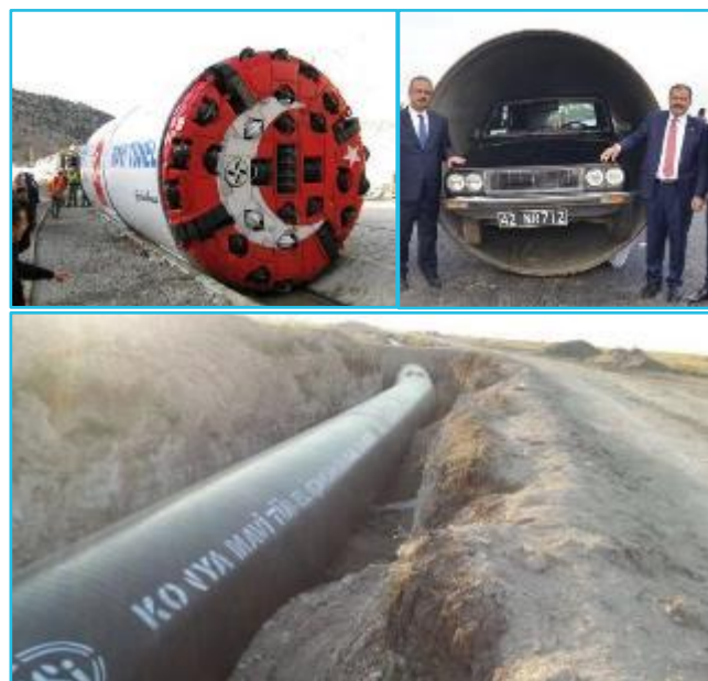
Image 39: The “Blue Tunnel Project”
