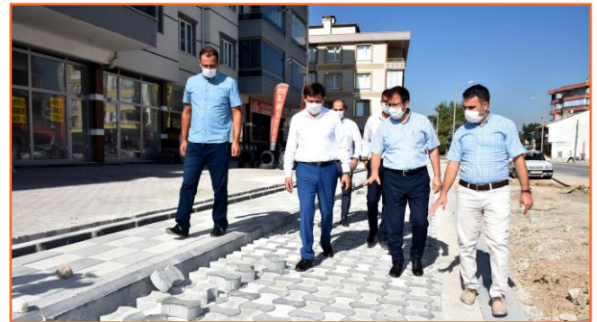
Image 54: Kerbs installation works in Karatay
