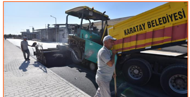
Image 55: Paving works in Karatay
