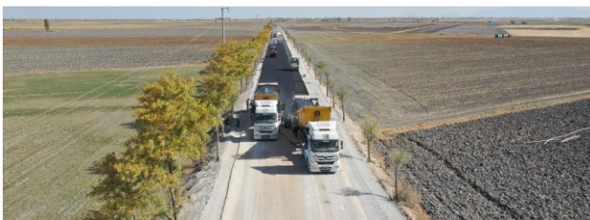
Image 10: Asphalt constructions in the suburbs of Karatay
