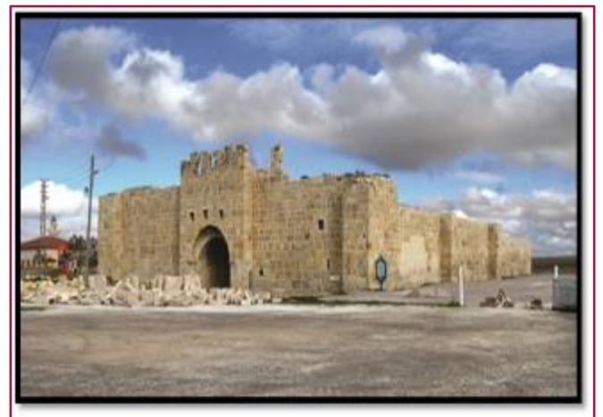
Image 51: Restoration of Obruk Inn
