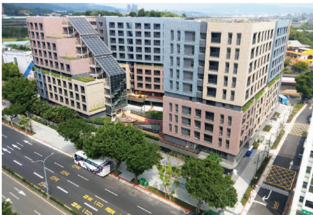
▲ Construct diversified social housing - Minglun Social Housing
