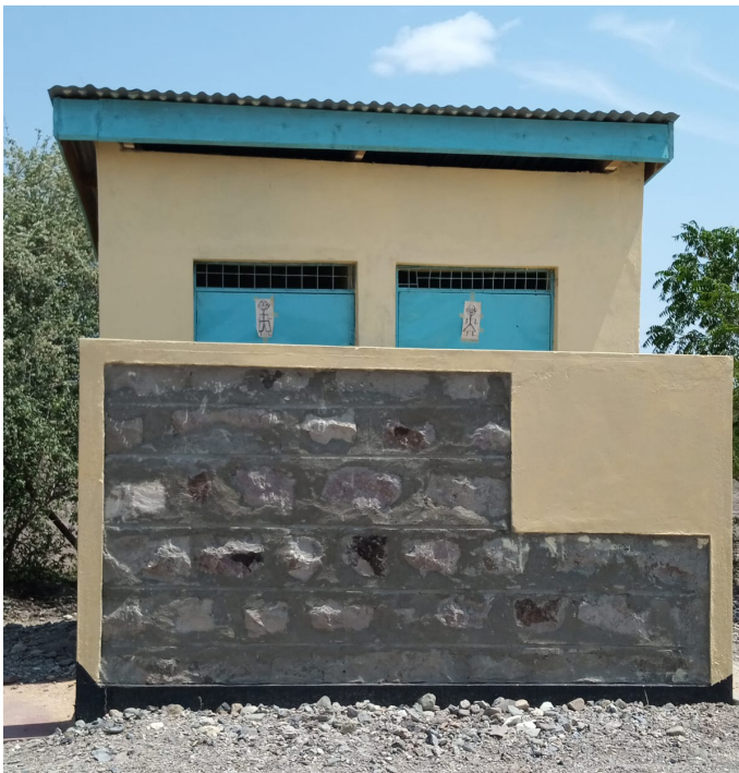
The two door pit latrine constructed at the KSCC. © UN-Habitat
