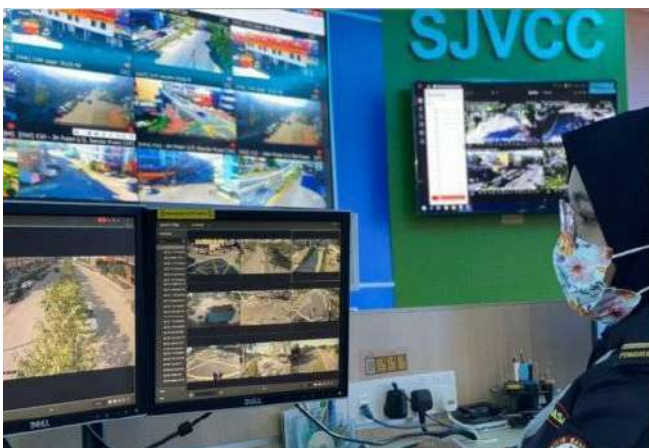
Subang Jaya Vibrant Command Centre
