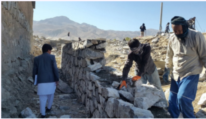
Construction of flood canal by community members in Kabul. © UN-Habitat Afghanistan
